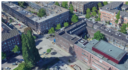
Figure 5.6: Example of a Magic Mix in a residential area: Baak Zuid (Gemeente Amsterdam, n.d.)
