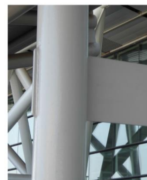
Figure 5: Example of a through plate connection to a CHS [6]
