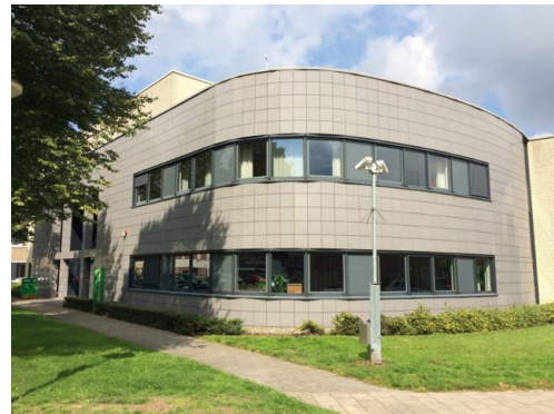
(a) Southeast view of building D
