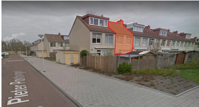
Figure 73 Build Type - Between Row House from (Google Maps, no date)
