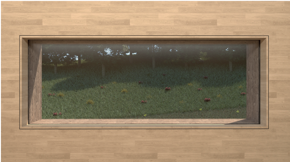
Figure 59: Window frames hidden behind fir element
