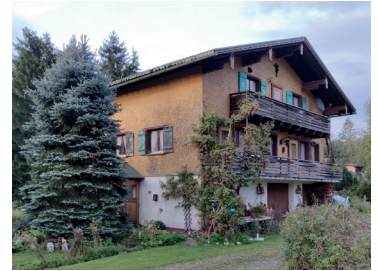
Figure 36: Austria typical house
