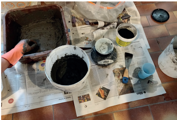
Figure 62: Mixing cement, sand, water and pigment
