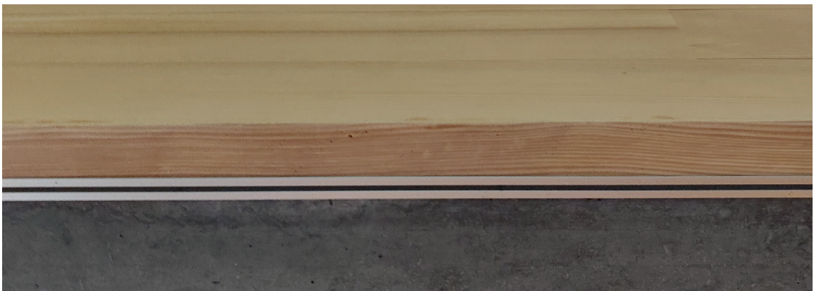
Figure 50: Curtain rail in the living room
