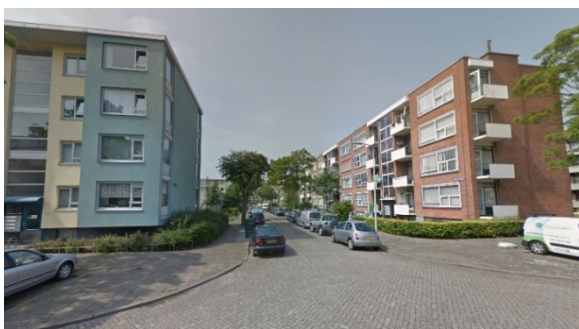
Figure 5.3: Cross between the Groenezijde and the Noorderzijde in Bouwlust / Vrederust. Typical 4 level apartment complexes (Google maps, 2019)
