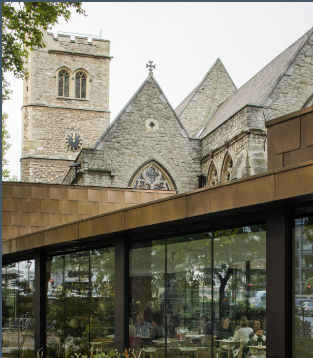
Figure 6: The Garden Museum's extension to the old church of St. Mary (Coleman, n.d.)
