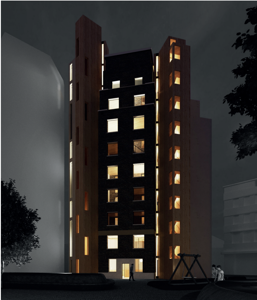
Figure 37: Light as a buffer between old and new
