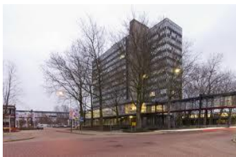
Figure 4: Building 1, Potentiaal (Europaan, 2014)
