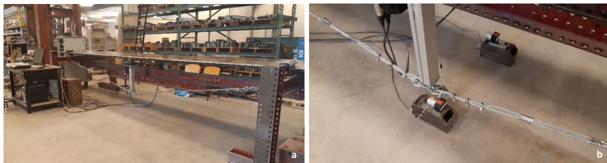
Figure 6.5: Pedestrian bridge with cable truss \varnothing 10 steel wires (a) and measurement devices (b)
