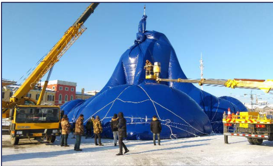
Figure 151; Connection of the rope net
