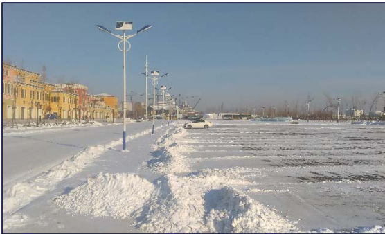
Figure 131; Building site is cleaned from snow
