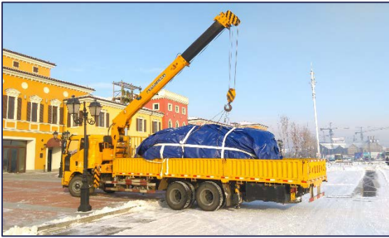
Figure 144; Arrival of inflatable on building site
