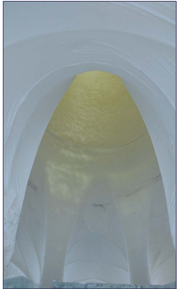
Figure 179; Inside of tower
