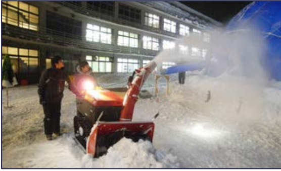
Figure 31; Application of snow on the inflatable source: (Kokawa, 2012)
