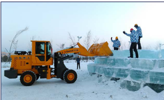
Figure 143; Stapling of ice blocks on fourth layer
