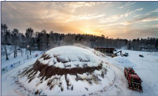
Figure 3; 'Pykrete dome' during construction; source: Bart van Overbeeke
