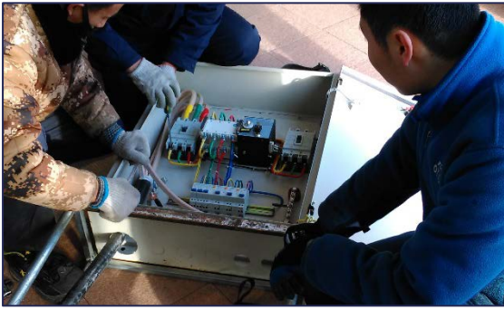
Figure 134; Installation of electrical cabinets
