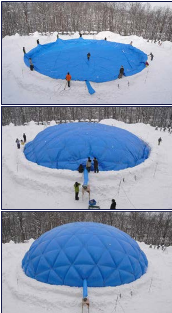
Figure 28-30; inflating the inflatable source: (Kokawa, et al., 2012)
