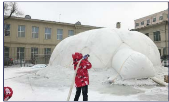
Figure 67; Spraying of test dome
