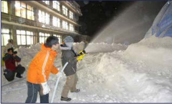
Figure 32; Spraying water on the inflatable (Kokawa, 2012)
