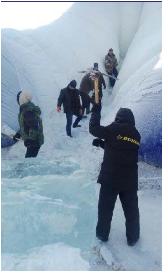
Figure 158; Addition of snow and ice between the legs the stimulate the shell development
