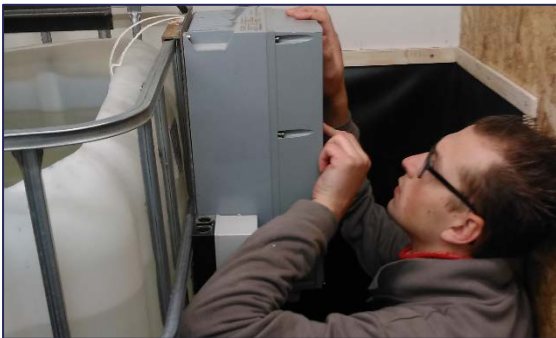
Figure 138; Installation and testing of the Cellcrete production line
