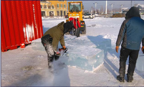
Figure 141; Modification of ice blocks by chainsaw
