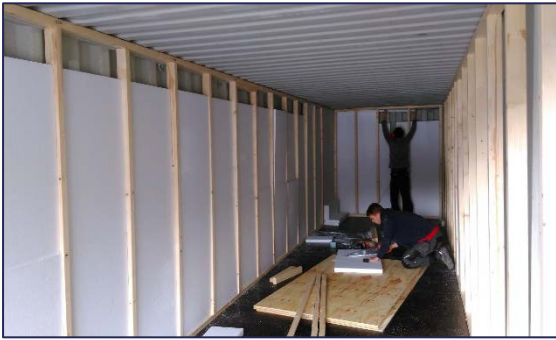
Figure 93; Construction of inner insulated wooden frame
