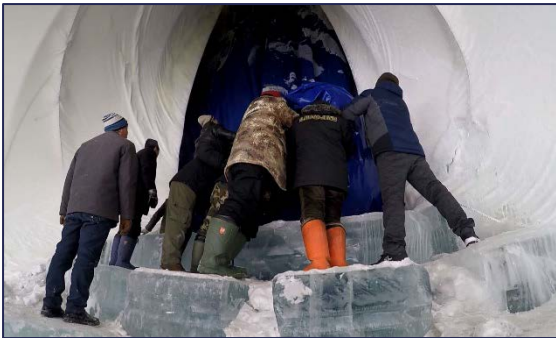
Figure 166; Removal of inflatable and pushing it inside
