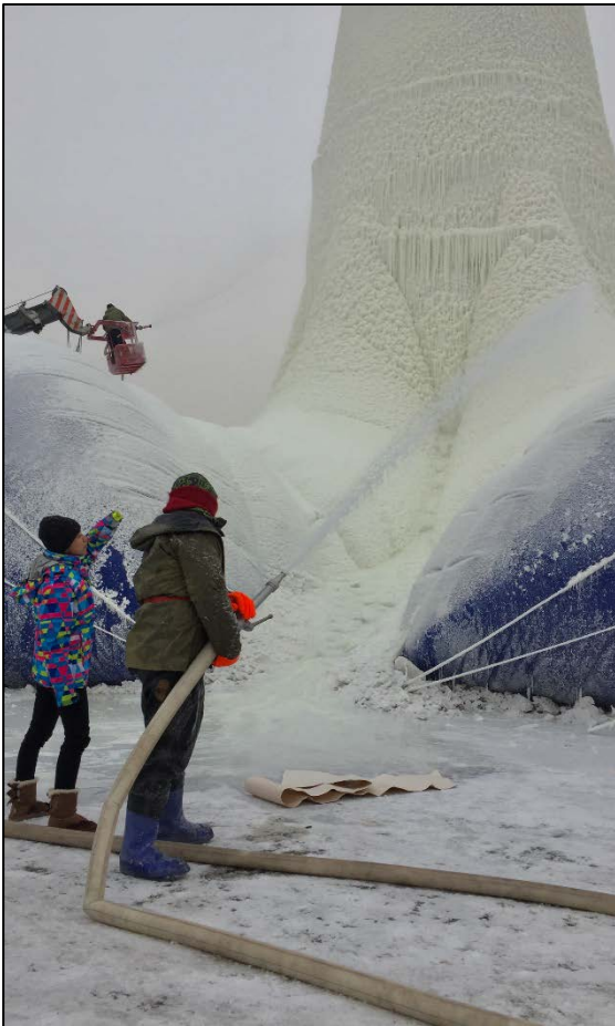
Figure 162; Spraying form boom lift and the ground
