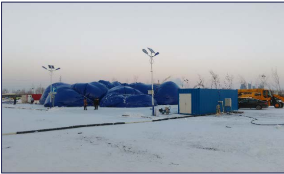
Figure 150; Minimal inflation of the legs
