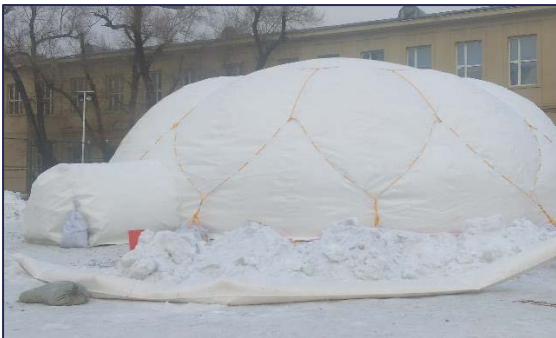
Figure 64; Inflation of test dome on building site
