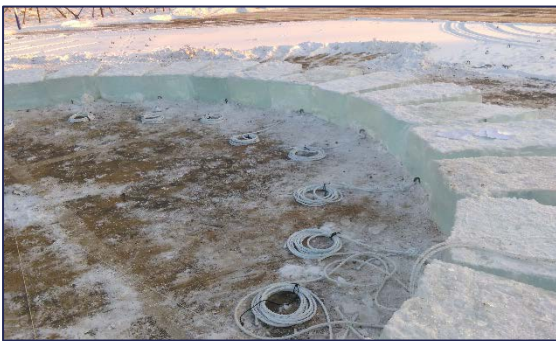
Figure 142; First layer of ice blocks with ropes attached to the middle anchors
