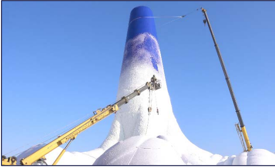
Figure 157; Spraying process of tower from boom lift
