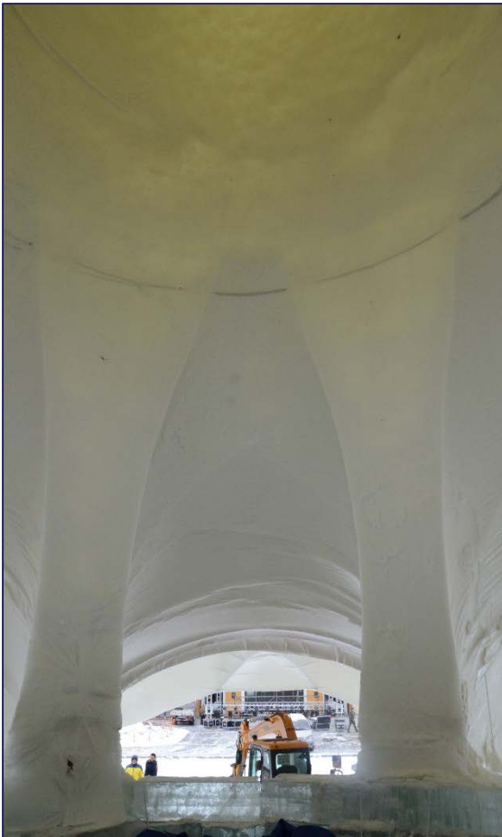
Figure 171; Finishing activities on the tower
