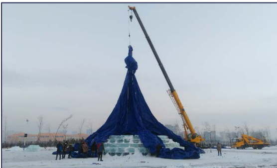
Figure 147; Hoisting inflatable in position
