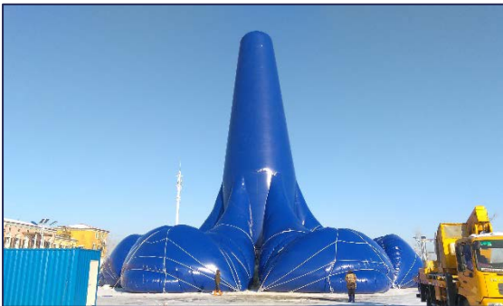
Figure 155; Full inflation after the untying of the top section
