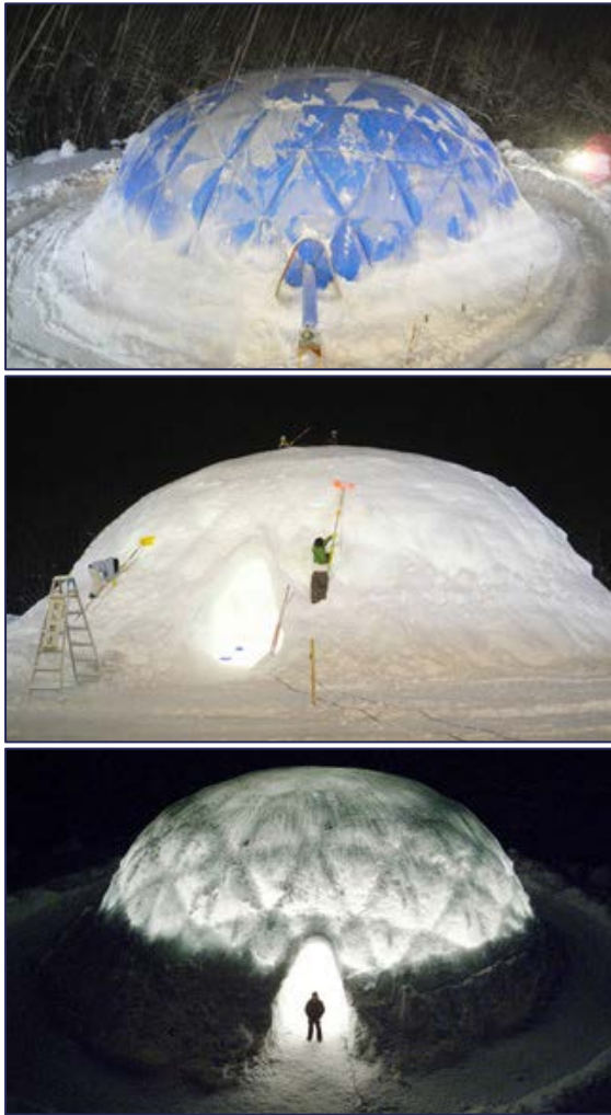
Figure 33-35; Removing of the inflatable; source: (Kokawa, et al., 2012)
