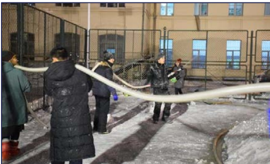
Figure 66; Crew handling the hoses for the spray process
