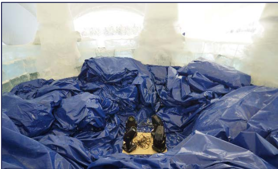
Figure 167; The inflatable is positioned in the middle
