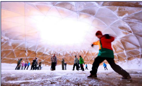
Figure 4; 'Pykrete dome' inside after completion; source: Bart van Overbeeke
