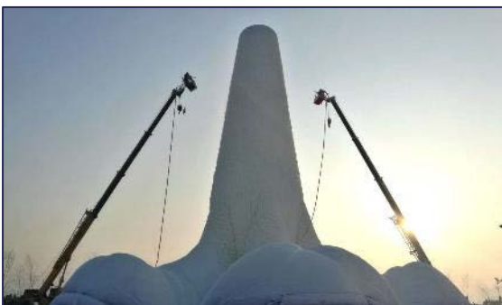
Figure 163; Spraying activities with two boom lifts
