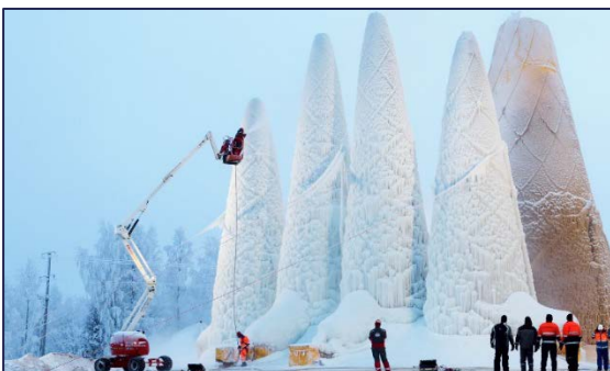
Figure 5; 'Sagrada in ice' during construction; source: (Kern, et al., 2015)
