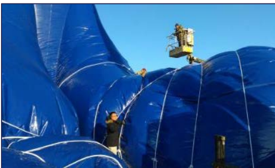
Figure 152; Connection of the rope net
