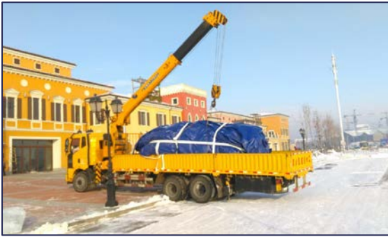
Figure 50; Folded and packed inflatable during arrival on the building site
