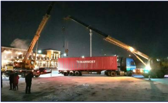
Figure 136; Positioning of Mobile factory
