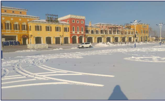
Figure 130; Building site in front of the Maple Leaf Village
