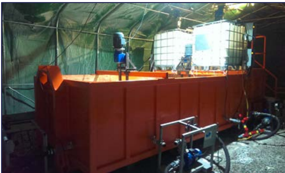
Figure 76; Overview of production line
