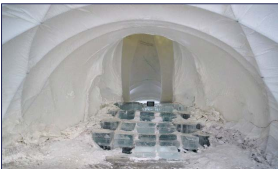
Figure 168; Ice stairs remain after the removal of the inflatable
