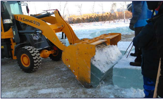
Figure 140; Stapling of ice blocks
