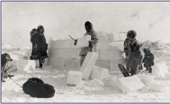
Figure 13; Eskimos building an igloo (Source: https://www.loc.gov/pictures/resource/cph.3c35985/ )
