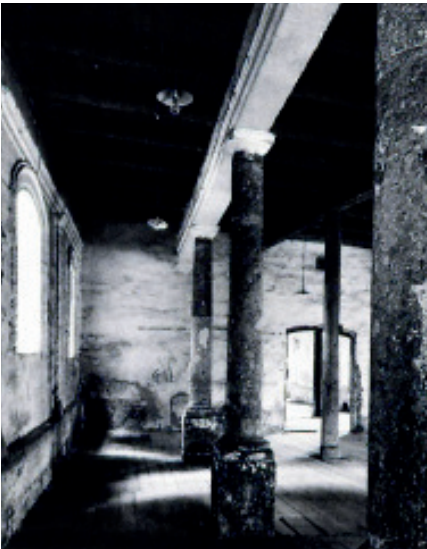
Interior along the wall of the first half, 1994
