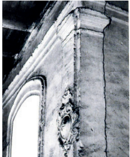
Ornamentation of stucco, 1994
