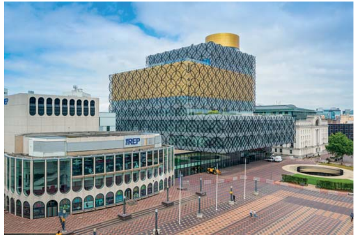
fig.2.36 The Repertory Theatre (REP) from 1960, The Library of Birmingham (LoB) and Baskerville House from 1936. © morrisroe.co.uk
