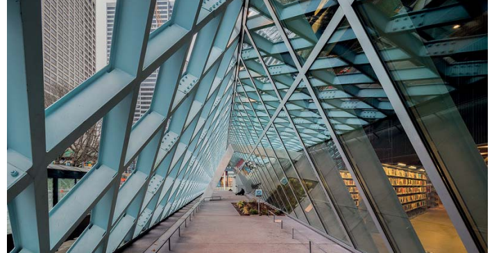
fig.2.9 Entrance "arcade" is an extension of the building's exoskeleton, and creates a seamless transition between the building and street. Photo © Darren Bradley
