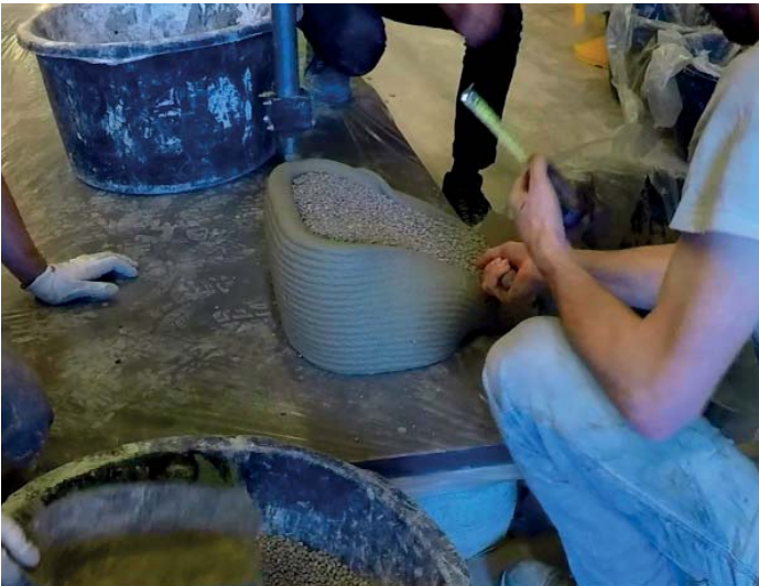
fig.1.4 Failed test - after filling layer by layer on the inside of the block without using the box, it fell after having printed about 20 layers.
