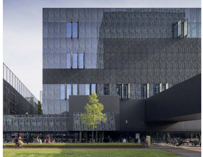
fig.2.25 View from the road side, with the main entrance in the plinth. The façade is covered with an abstracted image of fossilized papyrus printed on concrete panels, which are equal in size to the fritted glass panels. © archilovers.com
