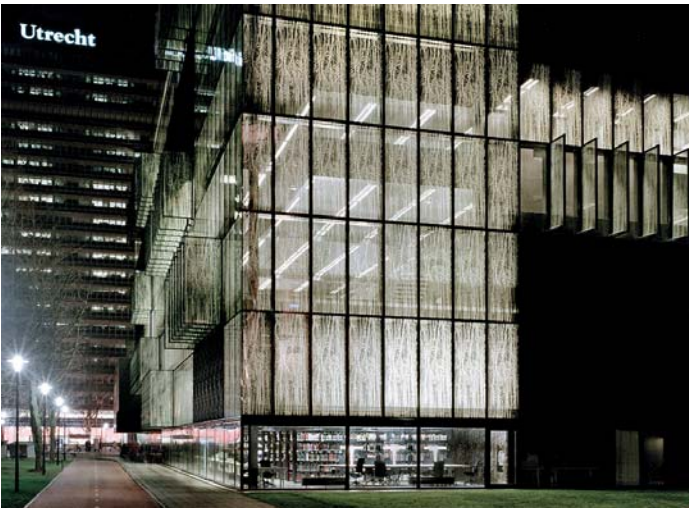
fig.2.23 The library at night with the printed glass and concrete panels. The light from inside to outside. © wielaretsarchitects.com
