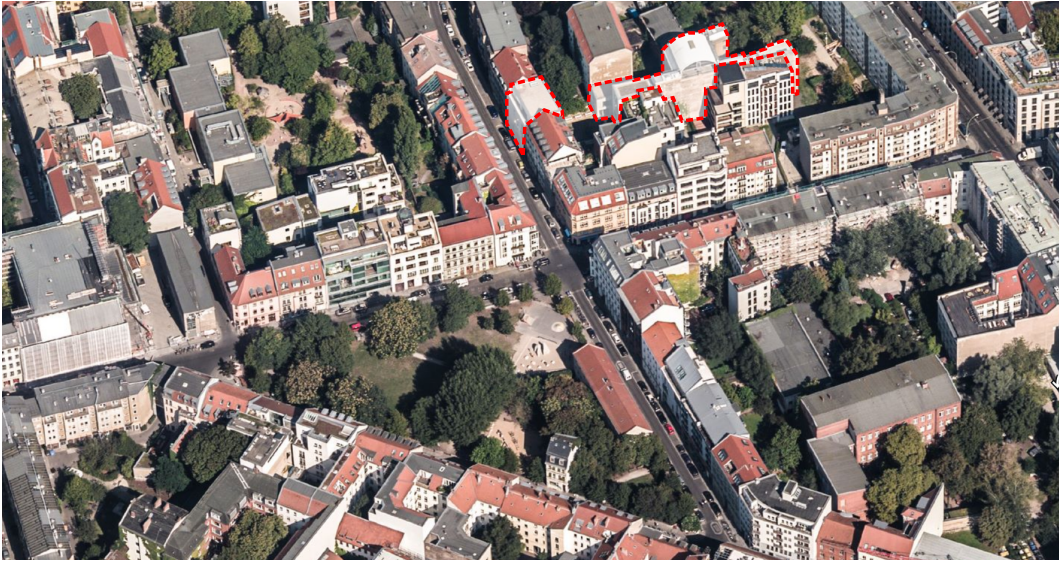
23. Birdseye view of the site Campus Joachimstraße is at the top north and is highlighted in red
