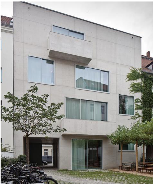
32. Front building's interior façade
