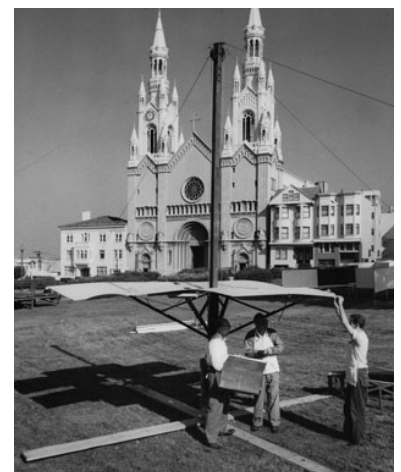
Figure I.3. The structure is supported by a central pole during construction.
