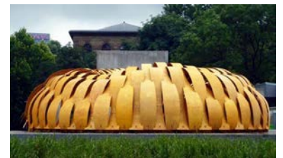
Figure III.1. The plate intersections are varied over the width of the structure.
