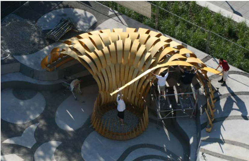
Figure 3.9. Assembly of the ICD/ITKE 2010 research pavilion (Fleischmann and Menges, 2011).
