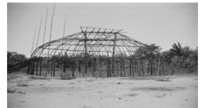
Figure 1.3. The Brazilian Oca house is a traditional bending-active structure
