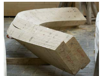
Figure 1.2. A double curved timber element from the Centre Pompidou in Metz.
