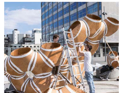
Figure IX.3. The modules are first closed before they are connected to each other.
