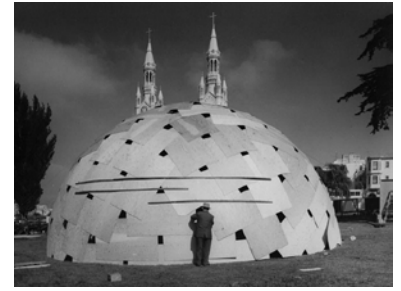
Figure 1.4. Plywood dome constructed by Thomas Moore in 1957 at Washington Square in San Francisco to a design of Buckminster Fuller.
