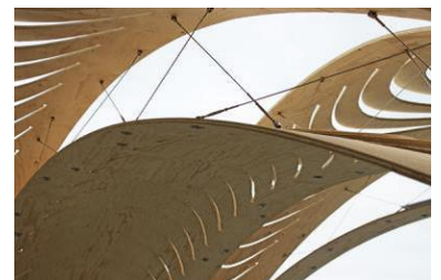
Figure 3.15. Tension elements in the AA/ETH pavilion (D'Acunto and Kotnik, 2013).
