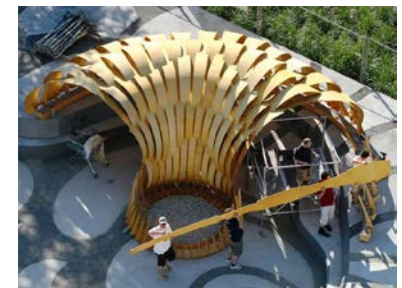
Figure III.3. Plywood strips are added one-by-one.
