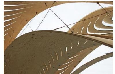
Figure V.2. The plates are connected by prestressed cables.
