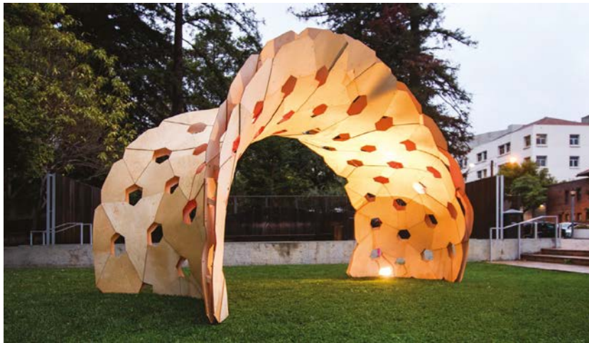
Figure 3.13. Bend9 project harnesses multi-directional bending to generate a double curved surface (Schleicher and Magna, 2016).
