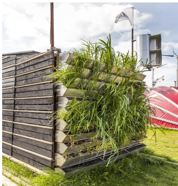
Figure 8: Tiny TIM purifying facade ( https://www.waterinnovatieprijs.nl/project/de-groene-wand-van-tiny-tim/ )
