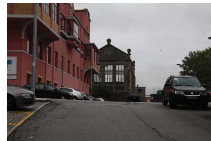
3. Entrance Rua de Sabrosa
