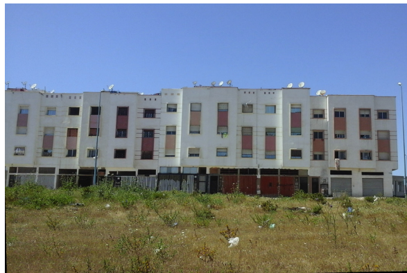
Figure 3.7: The new neighbourhood in Lahraouiyyine Source: Own work, April 2015
