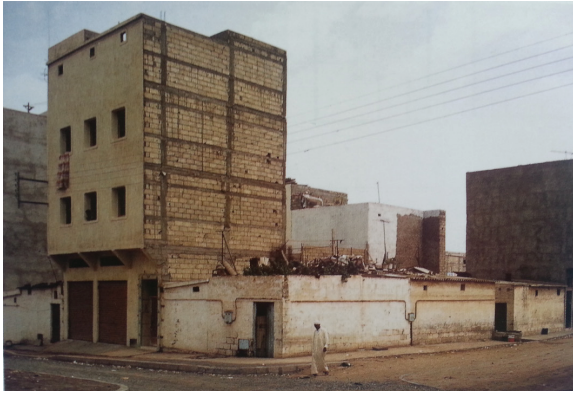
Figure 2.10: Vertical expansion of Cité Horizontale
