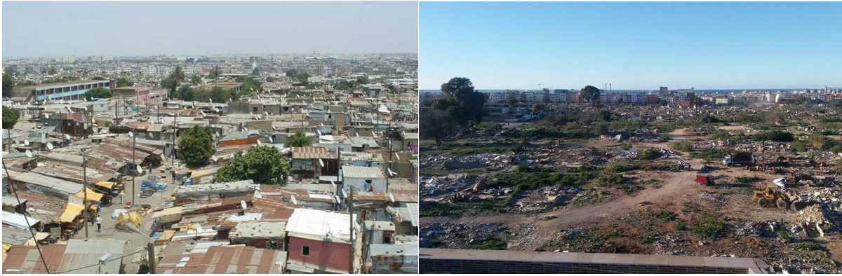
Figure 3.6: Carrières Centrales before and after demolition Source: Hay Mohammadi Facebook page
