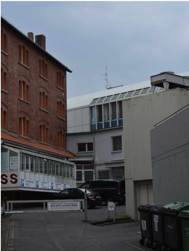
Fig. 50 Left on the image, industrial building now serves as a dance school
