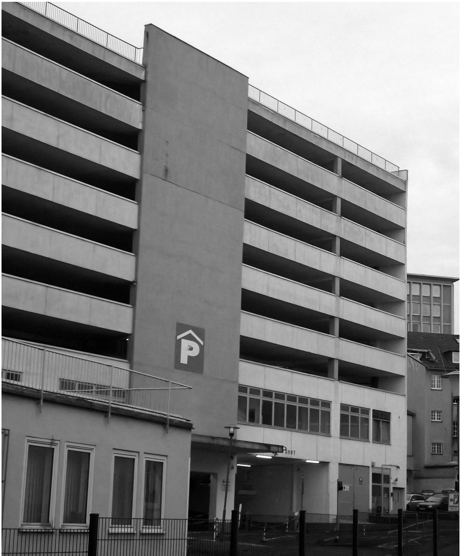
Fig. 16 Parking garage constructed in 1970, a repetition of floors which presents itself as a big block in its surroundings. Directly visible from the Königsplatz.
