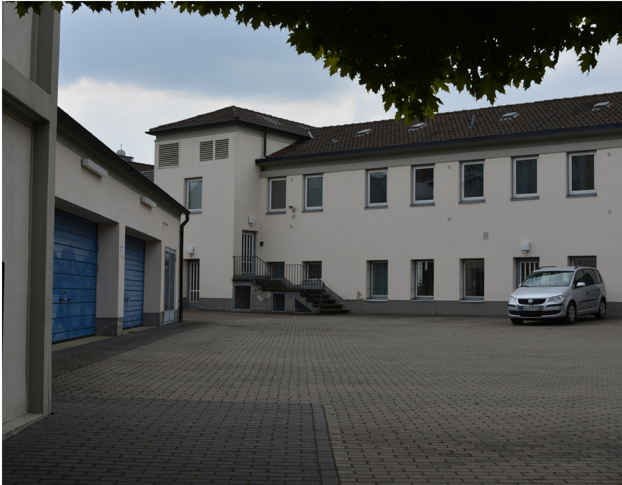
Fig. 61 View into the block with the parking garage left in the image.
