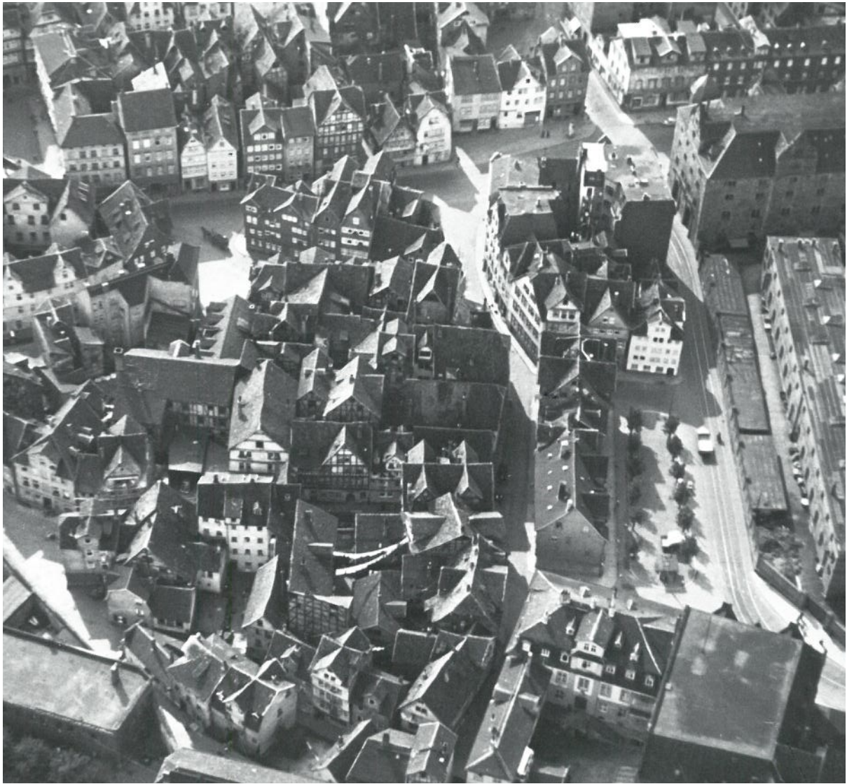
Fig. 28 Although fragmentation is often considered to be a characteristic of the modern city, the medieval city shows similar characteristic. The complexity of such a city fabric is overwhelming and can hardly be understood in terms of its design logics. Note the seemingly accidental characteristics of the buildings and the hybrid conditions of the urban spaces, often in-between what can be called a street or a square.
