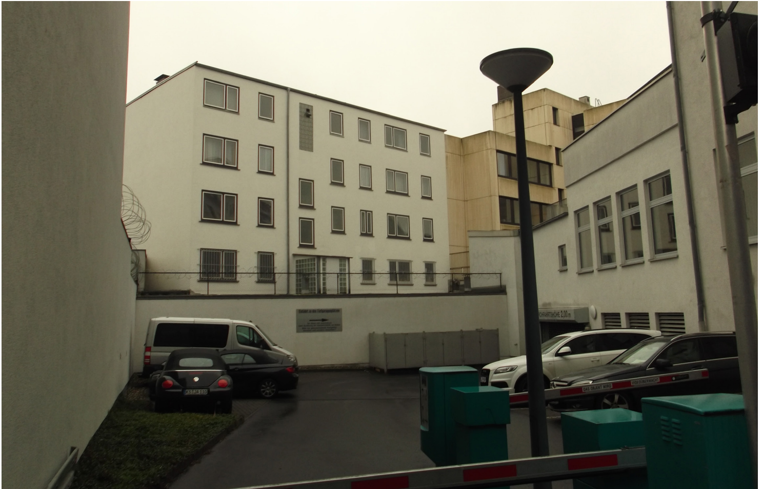
Fig. 55 closed off gap leading to parking garage
