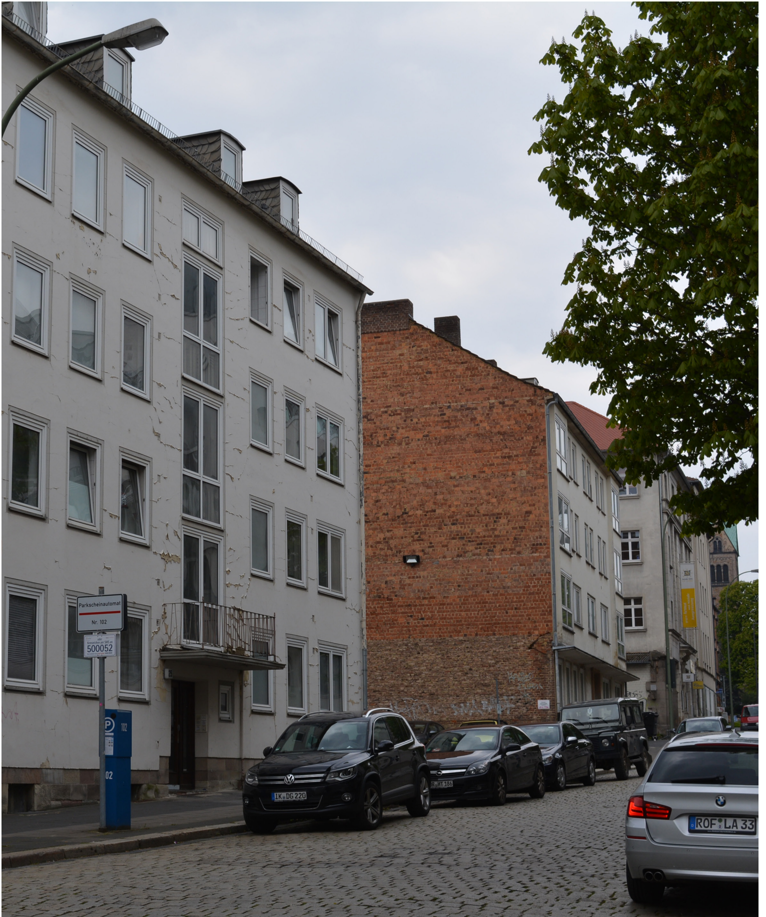
Fig. 20 A row of buildings that appears to be cut.
