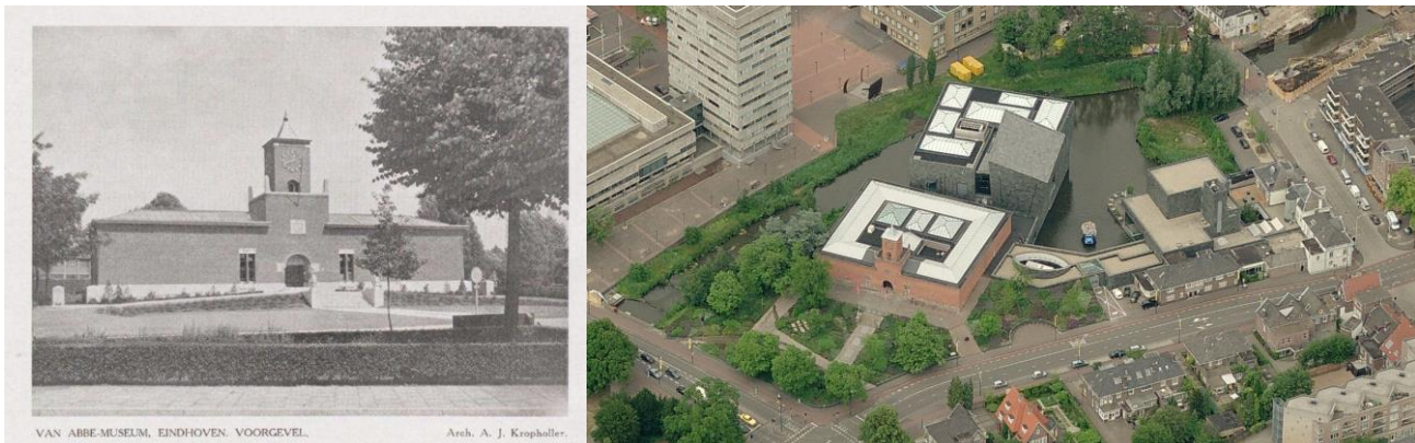
Figure 2.1: Left: front façade of the Van Abbemuseum in 1936 (Kropholler, 1936), right: bird's eye view (Bing Maps).
