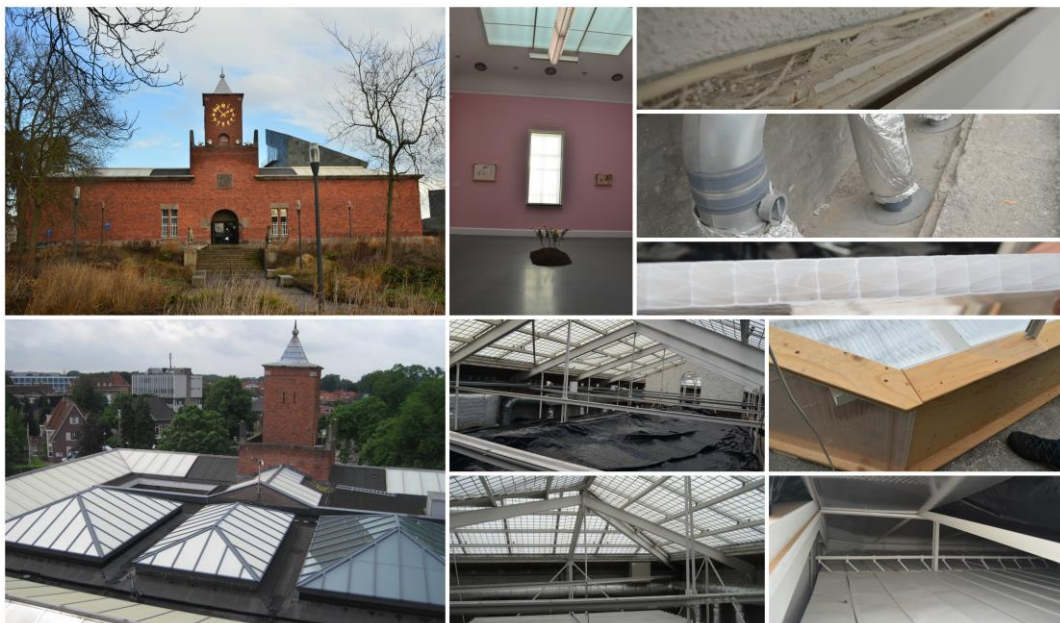
Figure 9.11: Structure types monumental building part A. South façade, interior exhibition room, double wall, plenum concrete, polycarbonate channel plate, roof view, plenums, polycarbonate channel plate structure covered with non-translucent plastic sheets above room 5.
