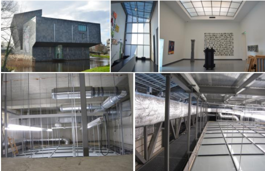
Figure 9.12: Structure types modern building part B. North and east façade, glass surfaces, interior exhibition room, plenum between floors, plenum below upper roof.
