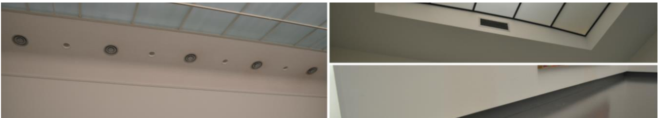
Figure 2.2: Inlets and outlets. Left: monumental building part A, right: modern building part B.
