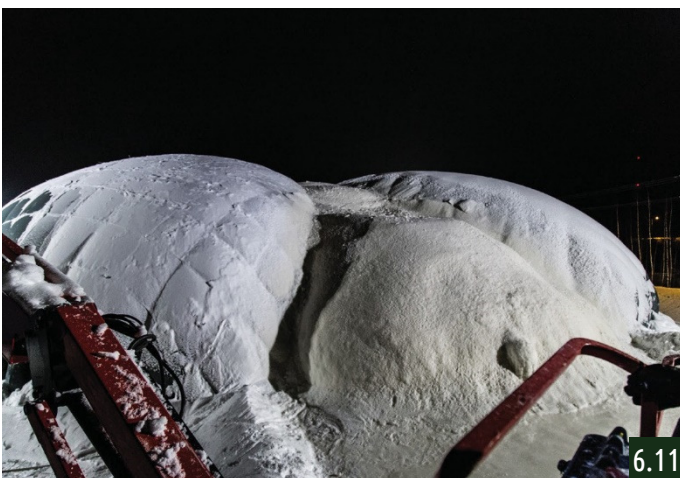
The sagged part resulted in a deformed arch, which was structural highly inappropriate
