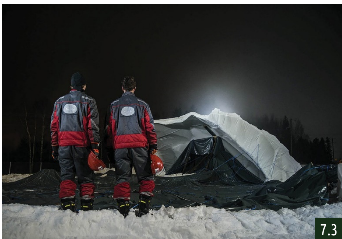
Unfortunately, in the very early morning of February 8, the balloon collapsed due to the warm weather. The constructed ice lost all its strength with these high temperatures
