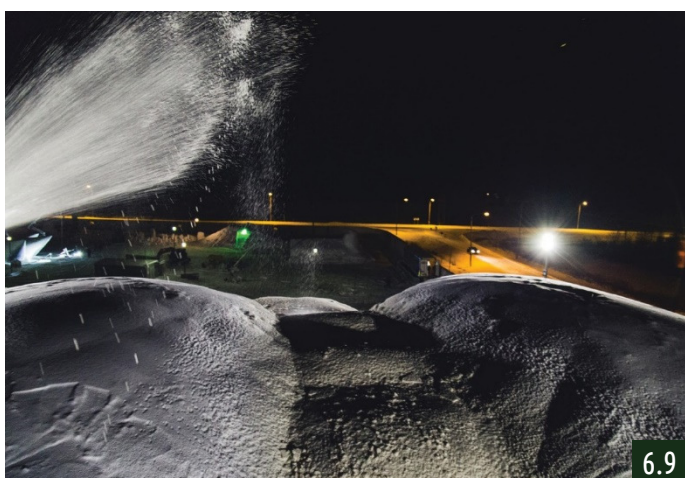
Trying to close the top part of the Bridge. You might notice the sagging of the Bridge at some points
