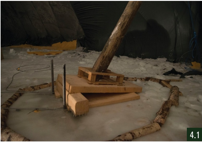
Feet of the columns are blocked by steel pins drilled into the ground, to prevent the columns from slipping away
