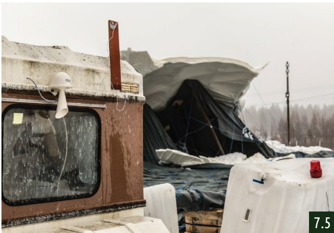
We were warned by alarms and flashing signs, and also by our monitoring system. This resulted in the fact that no one was injured during the collapse of the Bridge
