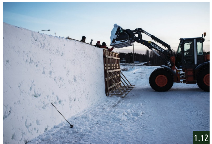
Finish volunteers created a huge wall of snow, to reduce the amount of fences we would need and to set up a cool snow area
