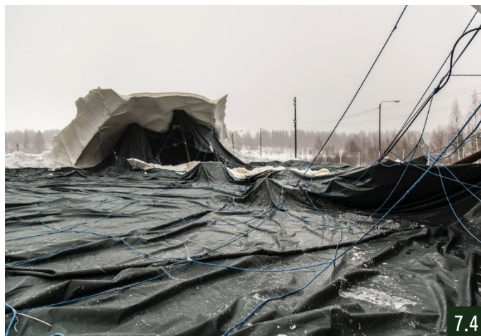
The inflatable was torn open over 25 meters. The feet of the Bridge, supported by the columns, held. They marked the imagination of how impressive the Bridge would have been.
