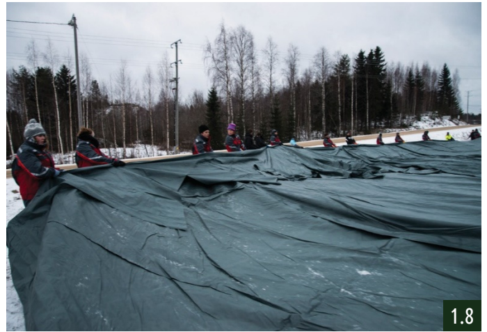
Pulling the inflatable in its exact position between the anchorpoints
