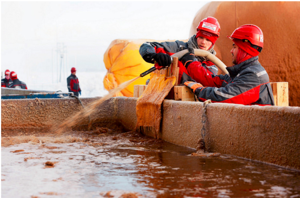
Figure 61: Frozen pykrete container during constructing the Sagrada Familia in Ice (Photo: Bart van Overbeeke)
