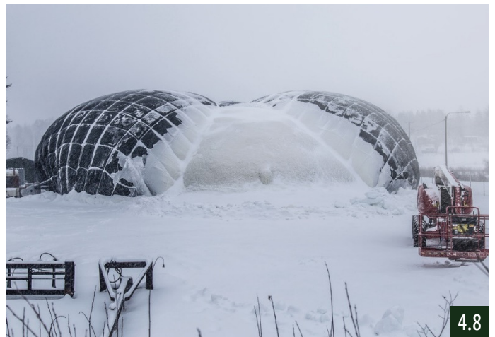
The bottom parts are fully sprayed, waiting for another cold period to connect them together and spray the top part of the bridge
