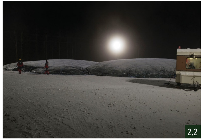
First volume of air inside the inflatable mold
