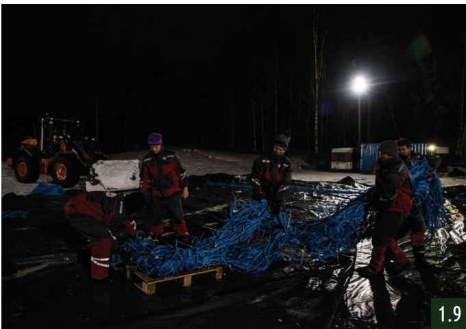
Unfolding the rope structure over the inflatable
