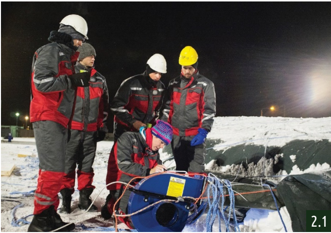
Connecting the air blower to the inflatable to start inflating
