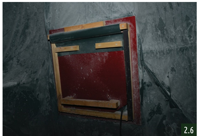
A created door in the balloon, to get inside the inflatable. By the internal pressure the door closed itself.
