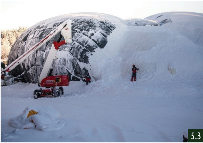
Removing snow from the Bridge and the inflatable, to reduce the carried load. In this week the temperatures were rising to almost 0 degrees Celsius, which occurred lots of trouble as leakage and heavy snow load
