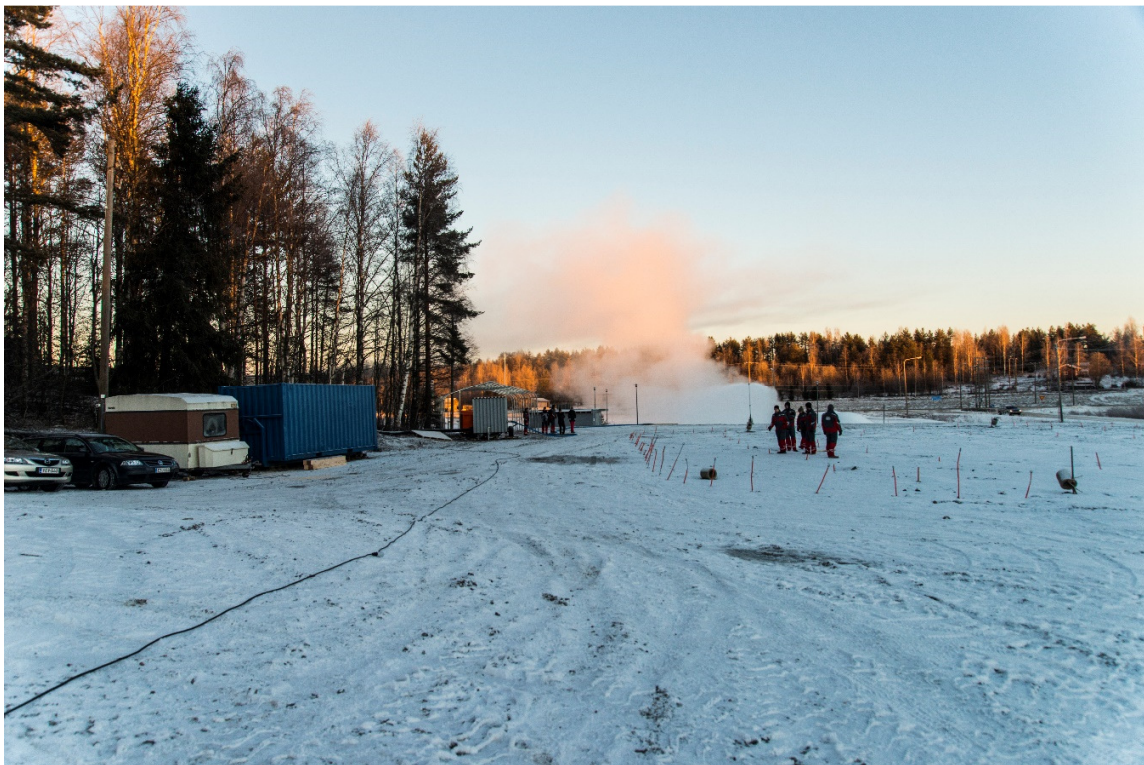
Figure 62: Overview of the building site at start of construction phase
