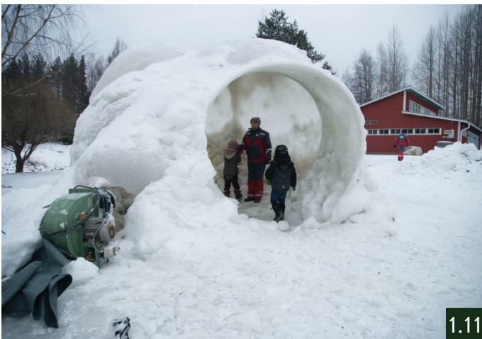
A side project; to get familiar with all techniques and materials we let volunteers practice with creating this 'bubble igloo'. This igloo is also made with an inflatable mold
