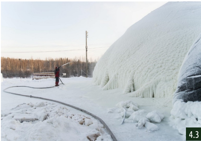
Spraying the mixture on the bottom part of the Bridge. Temperatures lay between -35 and -25 degrees Celsius this week.
