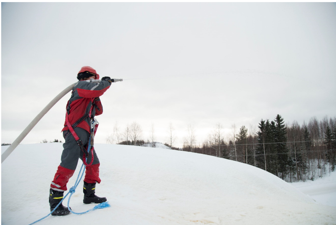
Figure 44: Working with safety helmets, gloves, working clothes and safety harness
