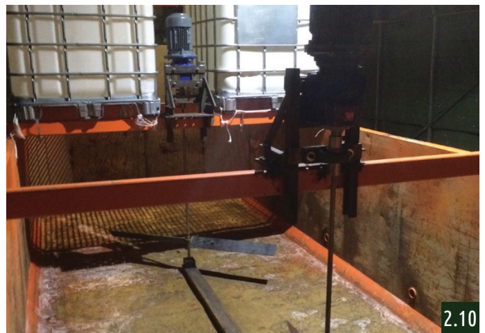
Installing the cellocrete mixing system
