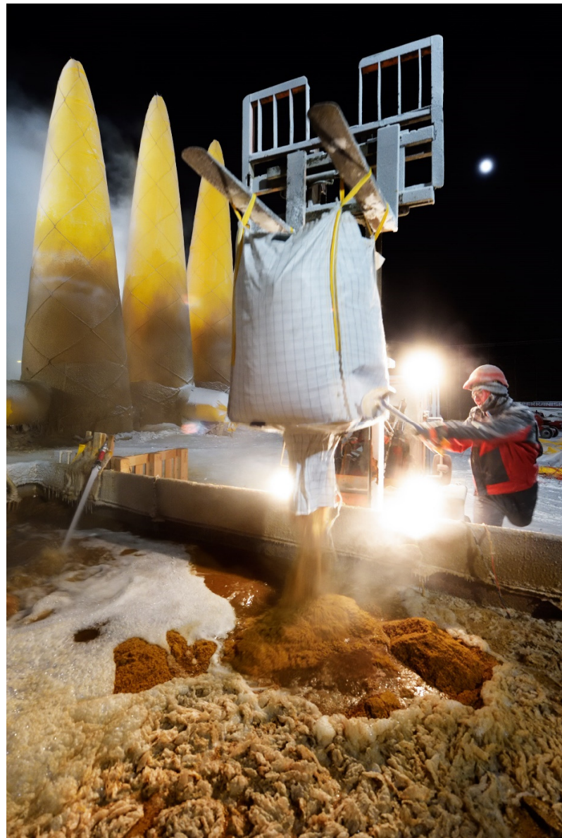
Figure 8: Mixing wooden fibers with water in a very improvised way during the Sagrada Familia in Ice project. (Photo: Bart van Overbeeke)
