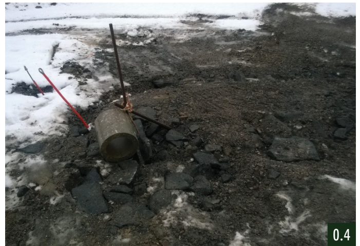
The four main anchors, placed at a depth of 2 meters
