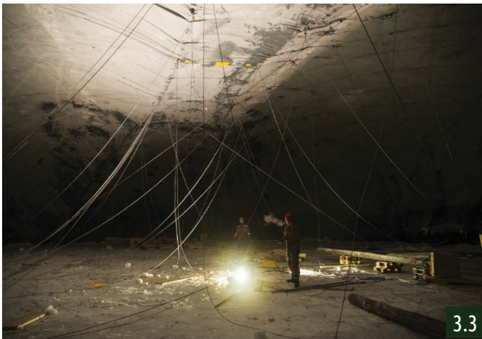
Steel cables for stabilizing just before tensioning
