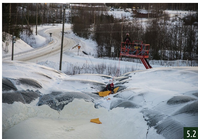
Another problem; the inside steel cables were tensioned to tight, occurring in a torn top part of the inflatable around the connection to the main cables. Again welding a new piece of foil was enough to save everything
