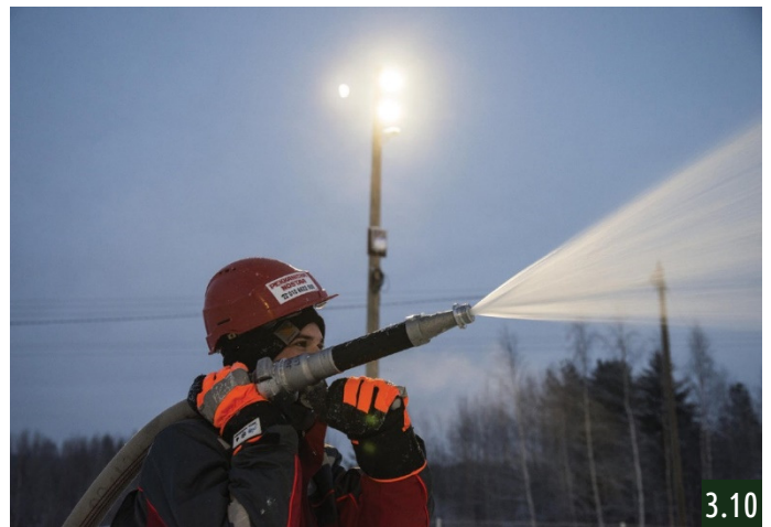
3.10 Volunteers spraying first layers of cellocrete on the inflatable mold
