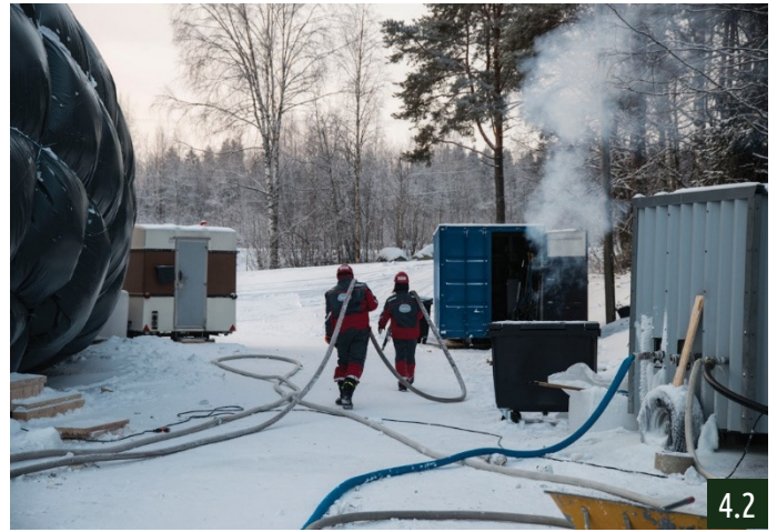
Volunteers moving the hoses to the other side of the Bridge, to continue spraying. On the right side the water house for pumping water from the quarry
