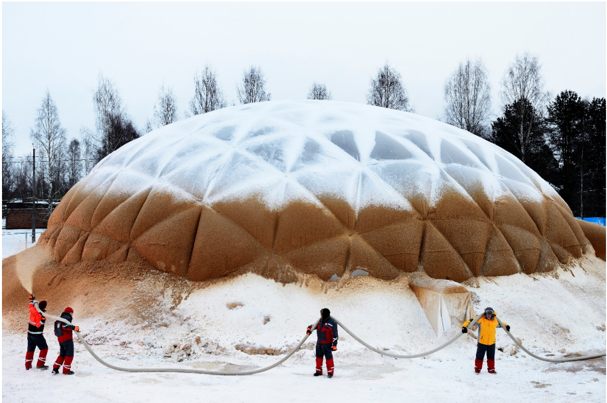
Figure 18: Pykrete dome under construction (Photo: Bart van Overbeeke)
