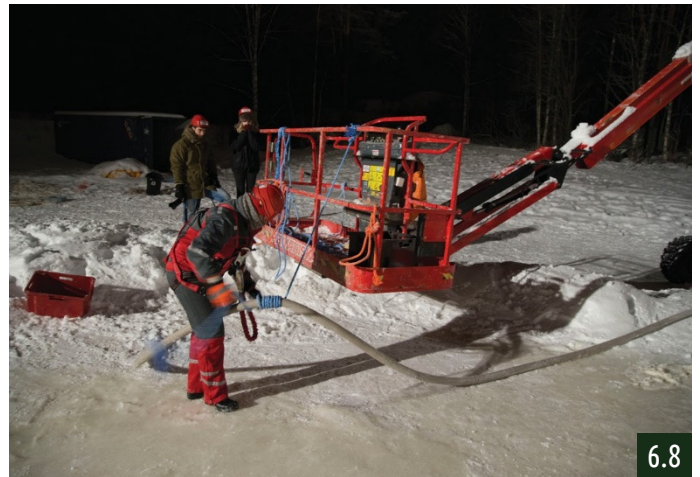
Start spraying again, with temperatures of -5 degrees Celsius it might be to warm, but with current weather forecast this might be our last chance to spray the top part of the Bridge
