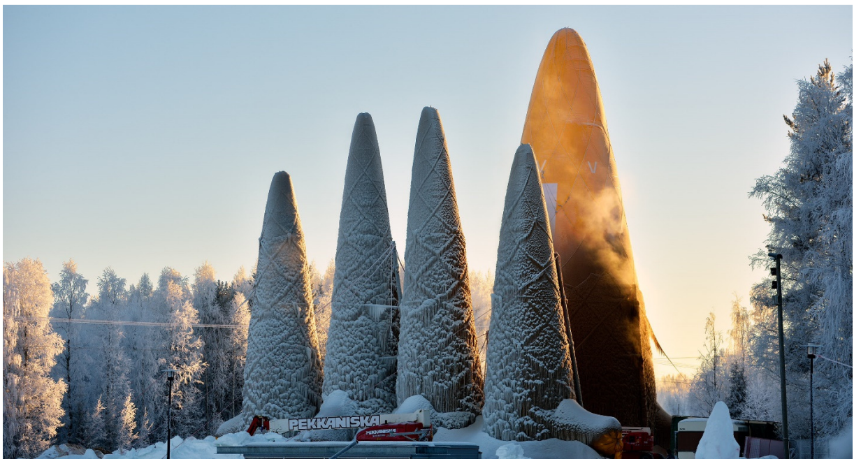
Figure 1: The Sagrada Familia in Ice project (Photo: Bart van Overbeeke)
