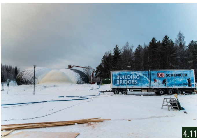
Overview of the building site. In the background the use of the boom lifts visible for the first time. Till than we could not use them because of temperature restrictions (only usable with temperatures above -23 degrees Celsius. In front a heated container.
