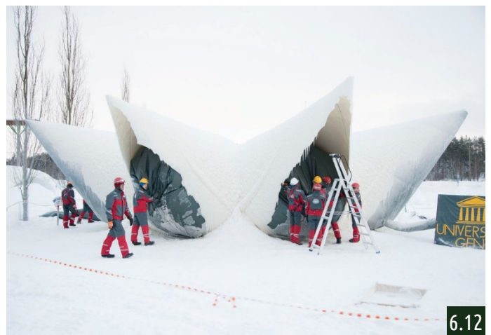
The inflatable of the Candela Pavilion deflated, with a thin ice shell as a result
