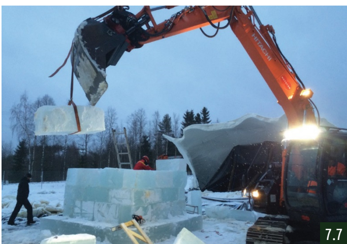
Creating a chimney of large ice blocks, cut from the Pielinen lake
