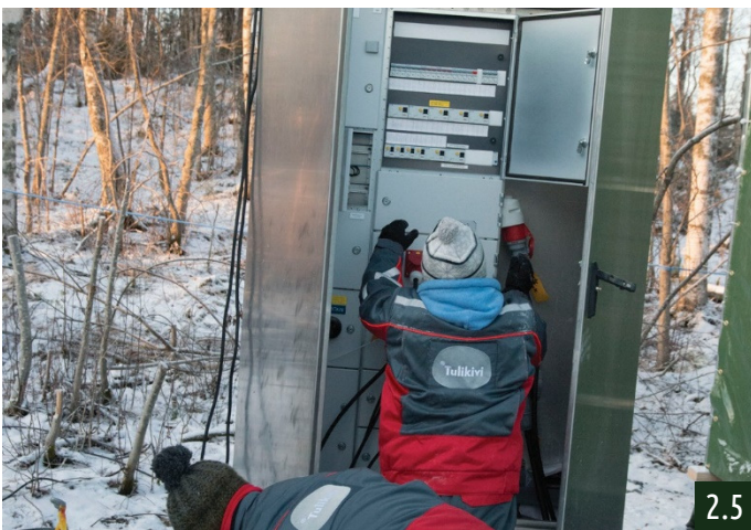
Connecting all prepared installations to the main cupboard on the building site
