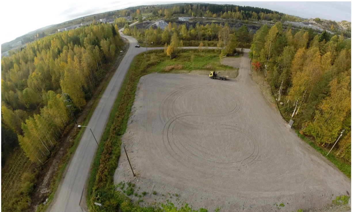
Figure 6: Building site during spring (Photo: Pentti Kalinen)
