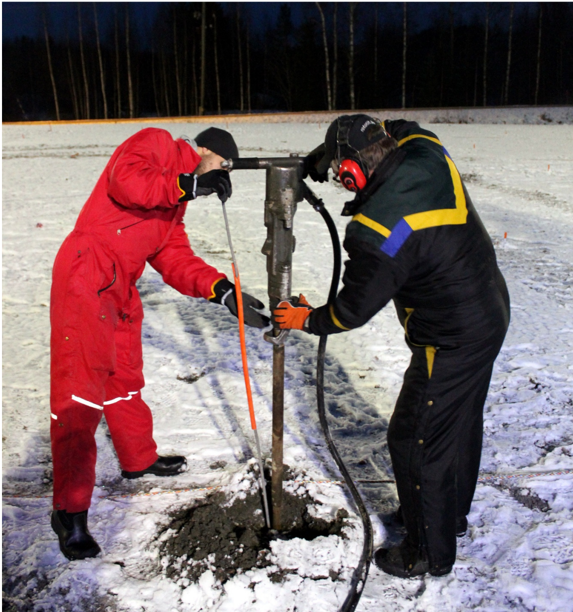
Figure 63: Drilling anchors
