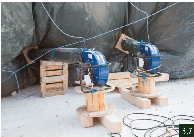
Final position of the air blowers and connected to the inflatable
