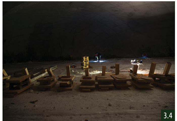
Prepared wooden parts for the extra supporting columns
