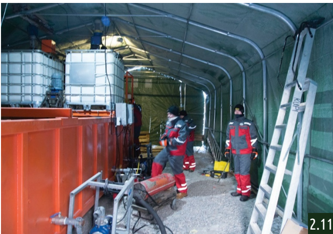
Connecting all pumps for distributing the cellocrete mixture to the inflatable, with the help of the Summa College students
