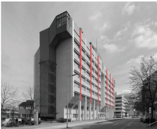
fig. 38 - Exterior installation services
