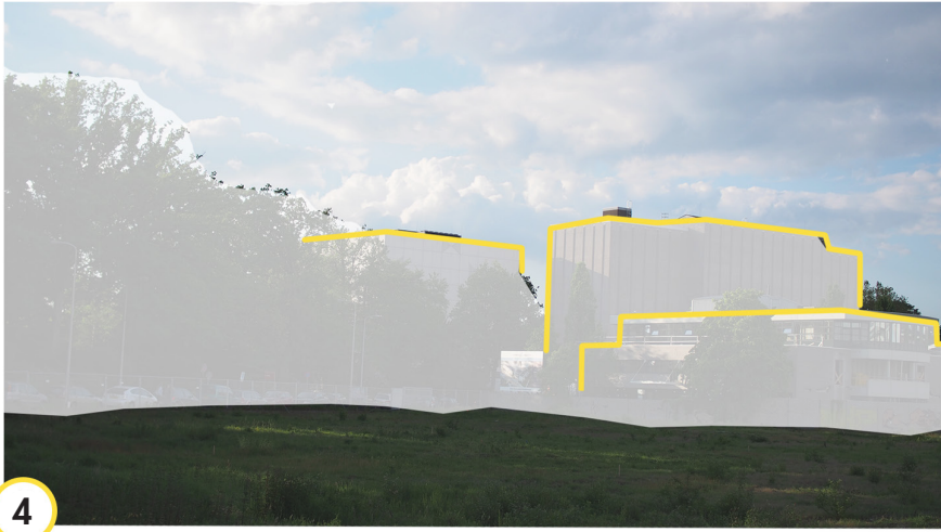
Figure 2.12 The edge of the park together with strong volume of the theatre.
