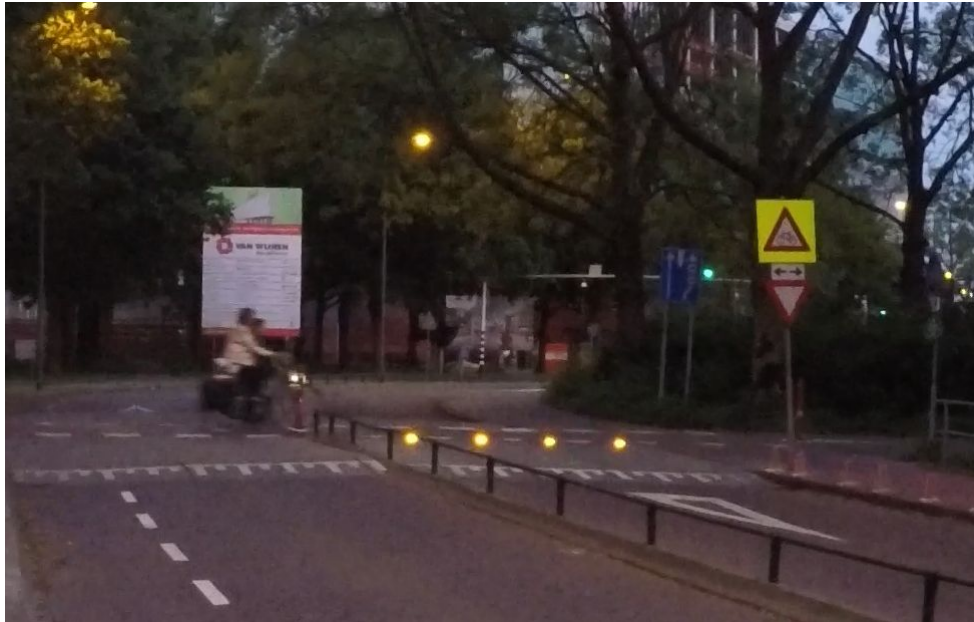
Figure 2.2. An example of in-pavement flash lighting system. Flash lighters are mounted on the road surface at a crossing for both the left and right lanes
