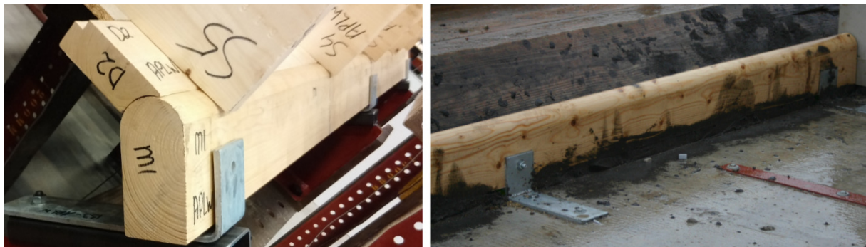
Figure 1.2b; Pictures of a typical round shaven wall plate
