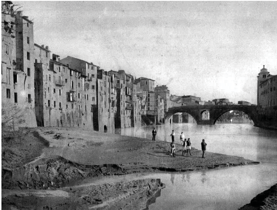
Fig.1 - The Tiber river before the embankment
