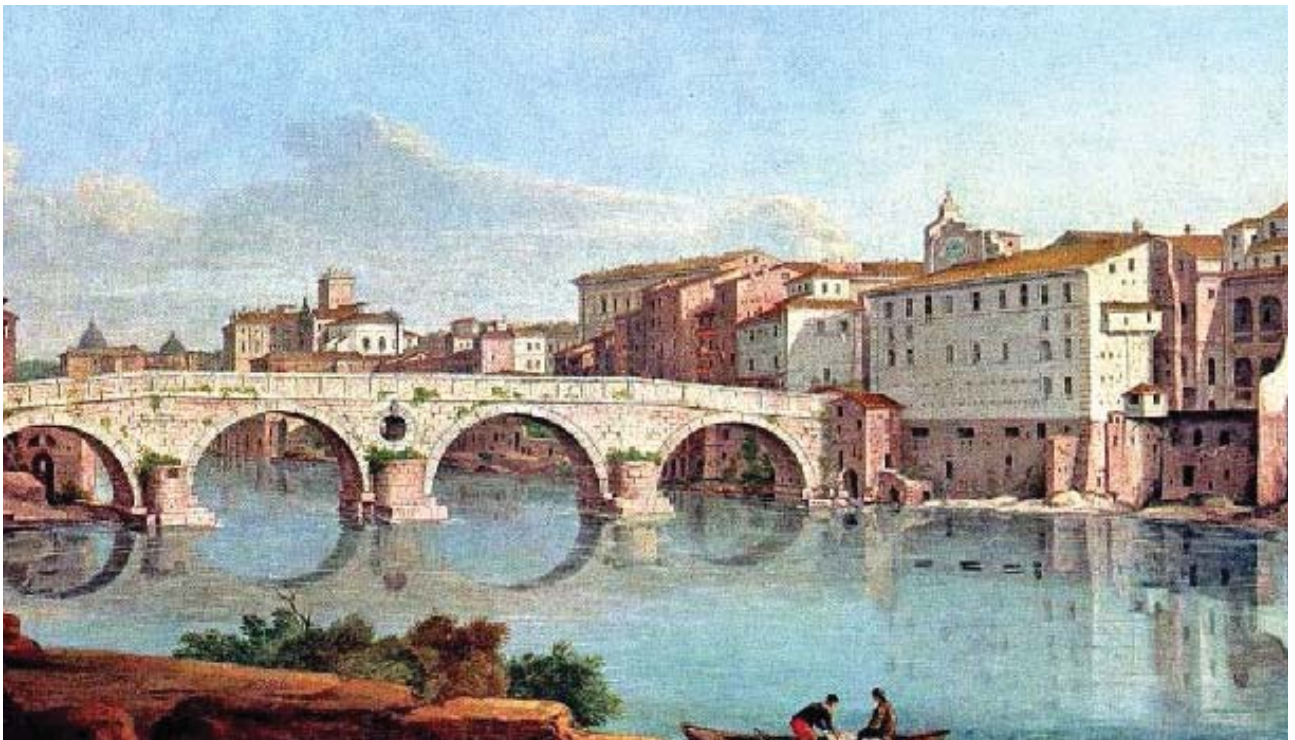
Fig.57 - Buildings that are founded on the river bed
