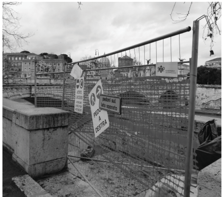
Fig.65 - Status of the stairs I
