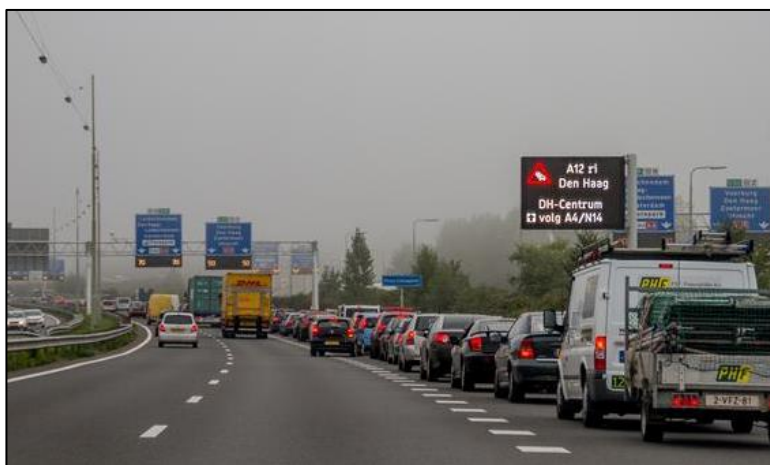
Figure 2 Dynamic sign (VMS) and the (blue) static signs background left. (Source: RWS-beeldbank 2013)
