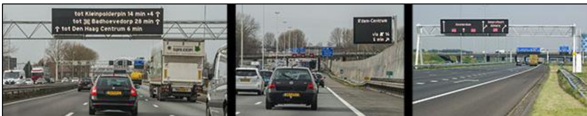
Figure 6 DRIP | bermDRIP | DRIP+ (Source: RWSbeeldbank | swarco.com)
