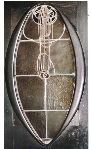
figure 31: leaded glass inserted in school doors
