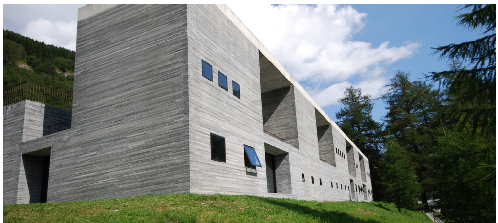
[39] Gevel Therme Vals
