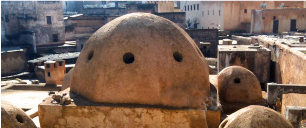
Fig. 13 – Roof structure with different light entrances
