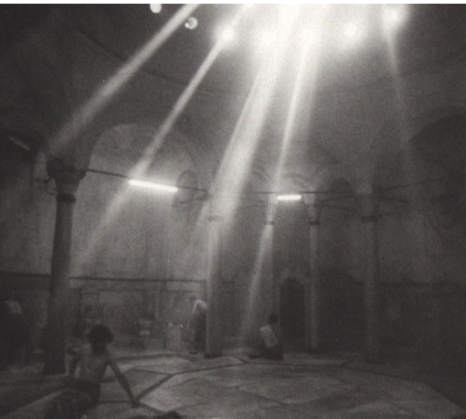
Fig. 23 – Light enters through roof light and small slots
