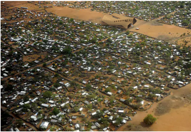
Fig 113. Building in Dadaab
