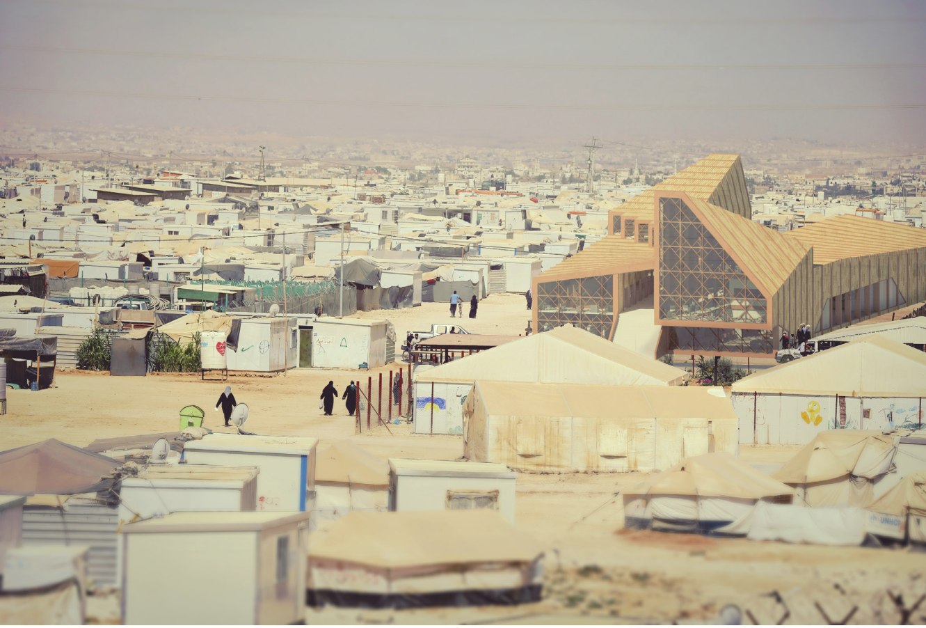
Fig 118. Building in the context of Za'atari
