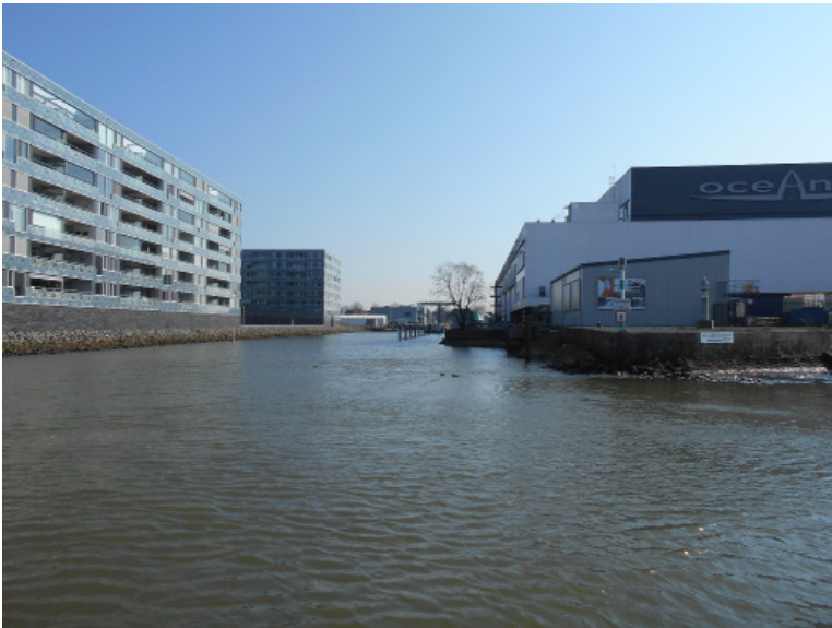
Fig 20: Entrance to city center via water and industrial building
