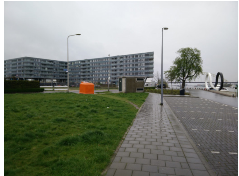
Fig 21 : Large residential building very close to the site
