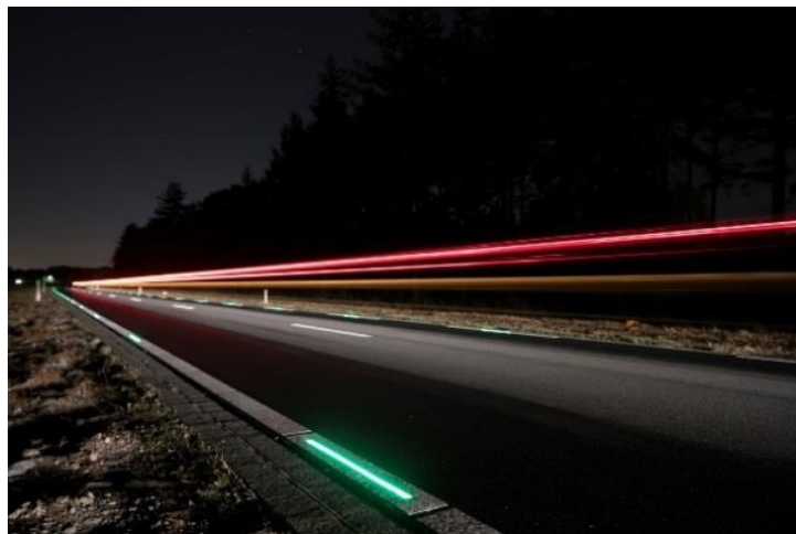
Figure 8: Light sources integrated in the road marking, activated with a green colour.
