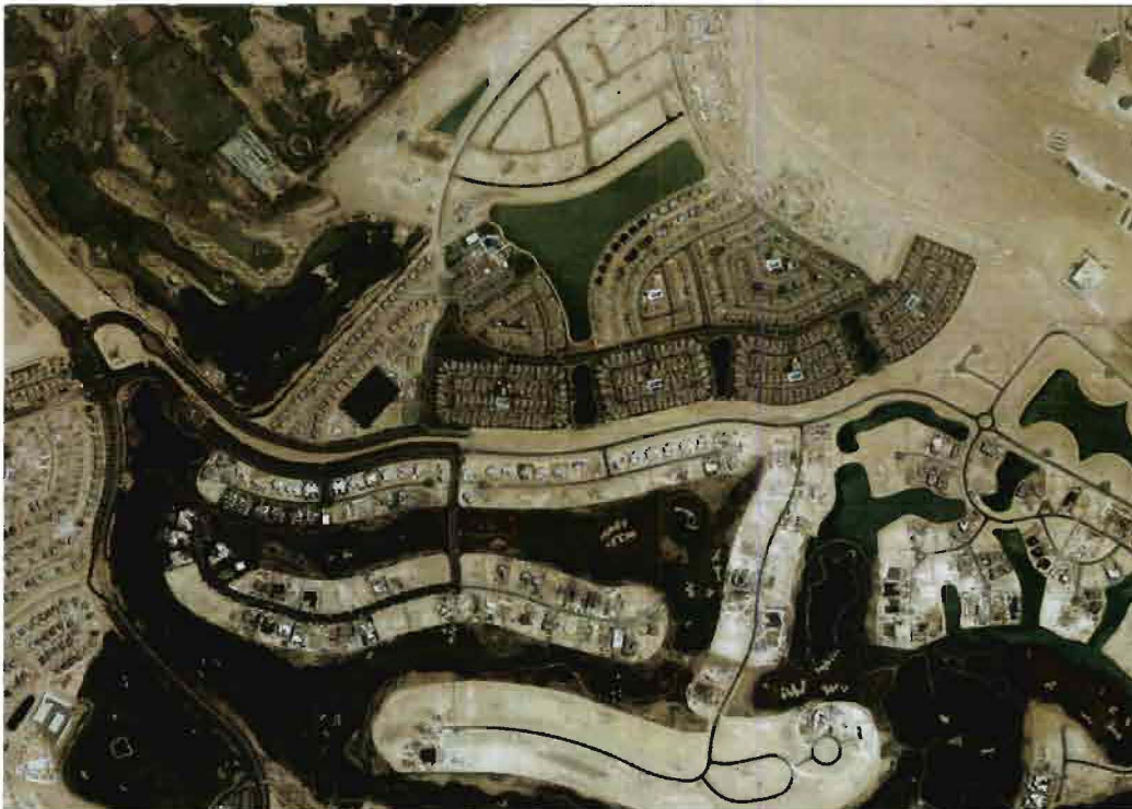
Photo 1: Aerial view gated community the Lakes under construction (source: UAE Locator)
