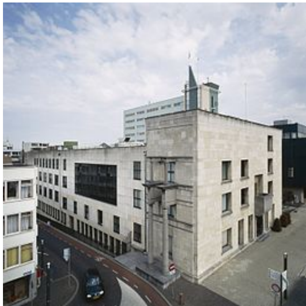
Figure 27 City Hall Heerlen
