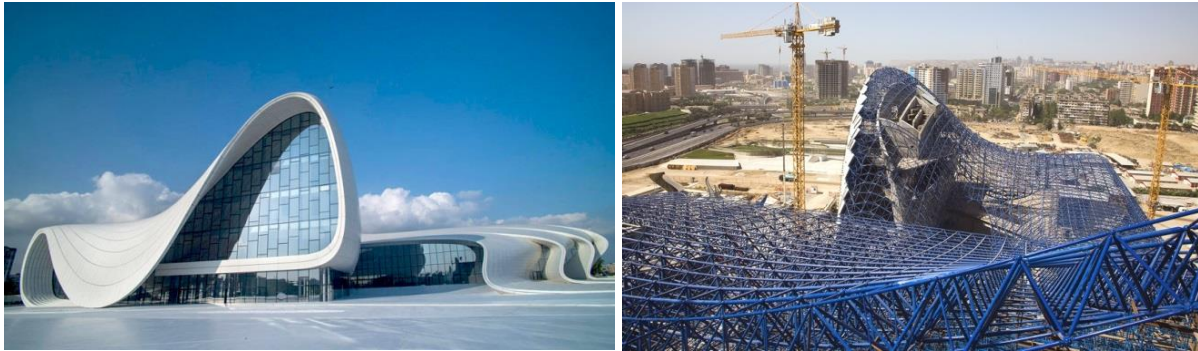
Figure 12a: Heyder Aliyev Centre (Designboom, 2013) & Figure 12b: Space frame of Heyder Aliyev Centre (Majid, 2013)
