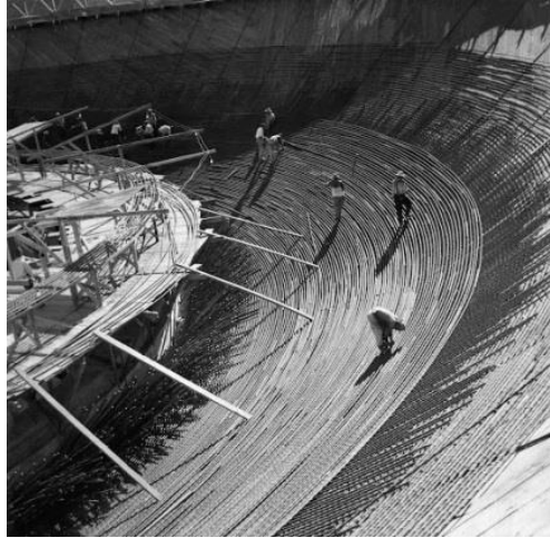
Figure 2: The construction of the National Congress in Brasilia (Cultural Institute, 2014)
