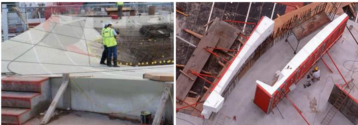
Figure 18a: EPS formwork of Spencer Dock Bridge (Huyghe & Schoofs, Precast Double Curved Concrete Panels, 2009) & Figure 18b: EPS fromwork of Der Neue Zollhoff (Janssen, 2011)
