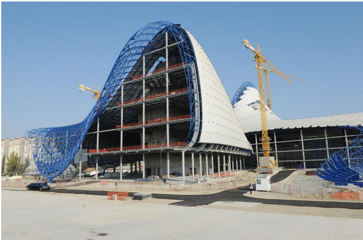
Figure 45: Construction of the Heydar Aliyev Center in Baku, Azerbaijan (Skyscrapercity.com, 2010)
