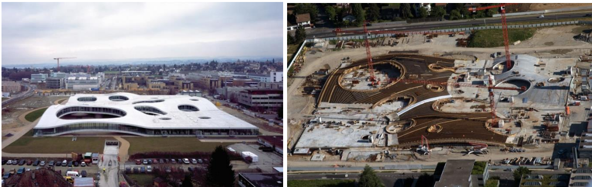
Figure 6a: Rolex Learning Centre (Eikongraphia, 2008) & Figure 6b: Rolex Learning Centre under construction (Busalto, 2013)
