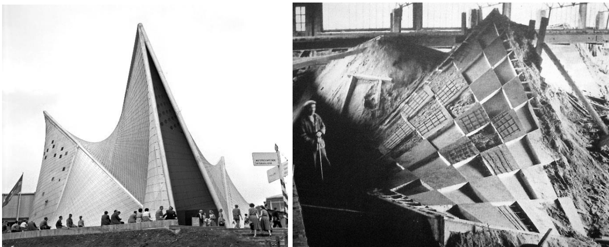
Figure 3a: Philips Pavilion (Wikipedia, 2014) & Figure 3b: Philips Pavilion under construction (McGill, n.d.)
