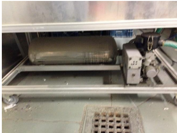
Figure 99a: Buffer tank to control the pressure & Figure 99b: Controller of the pressure
