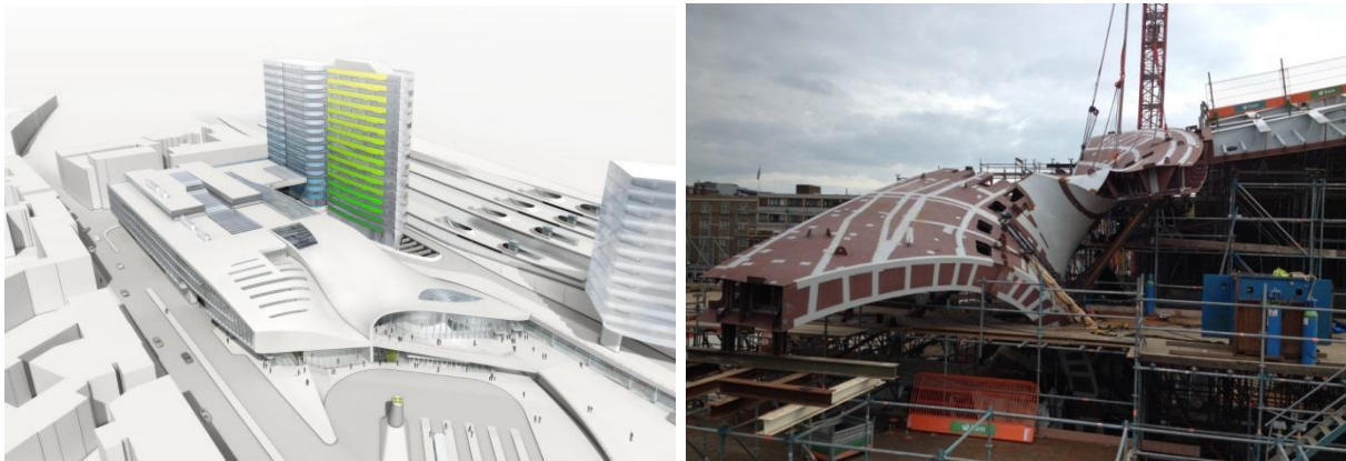
Figure 8a: OV-Terminal (Citypics.nl, n.d.) & Figure 8b: OV-Terminal under construction (Dibec, 2014)
