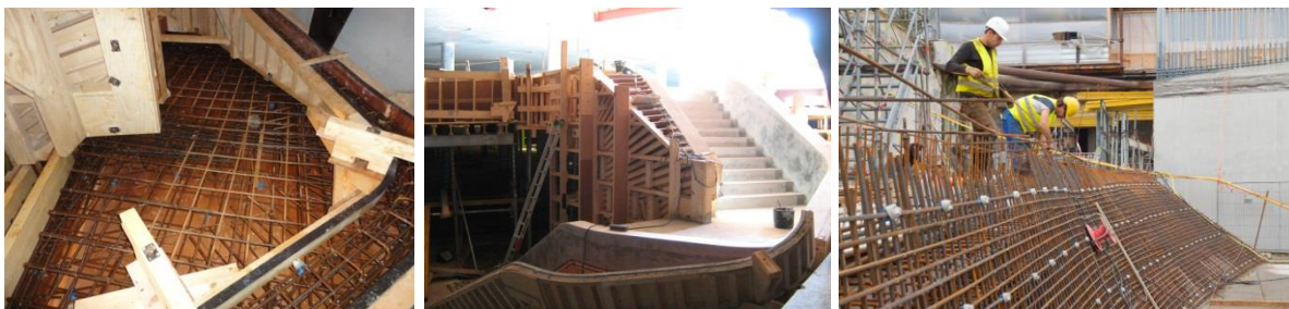
Figure 10a & 10b: Traditional wooden formwork & Figure 10c Reinforcement (Arnhem Centraal, 2010)
