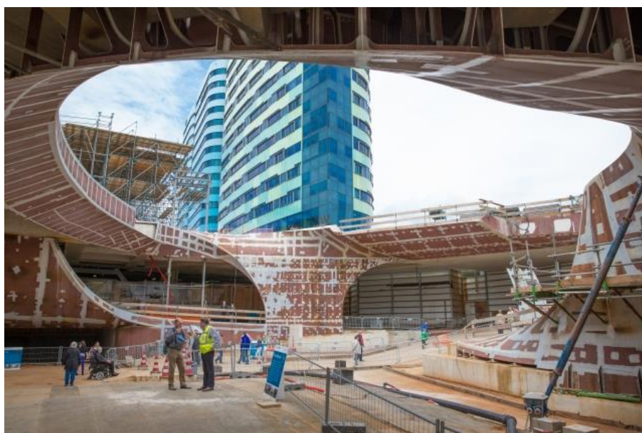
Figure 13: Inside steel structure of the OV-Terminal (Arnhem Centraal, 2014)
