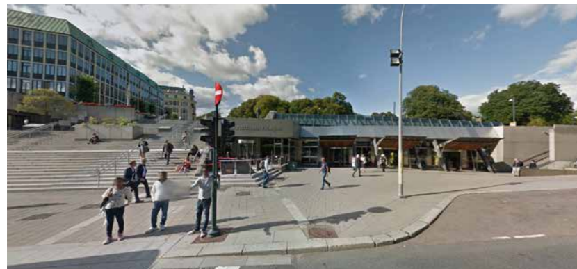
Fig. 22. Place of the 7 th June seen from the bottom of the monumental staircase. The main entrance of the metro station is made of three openings.
