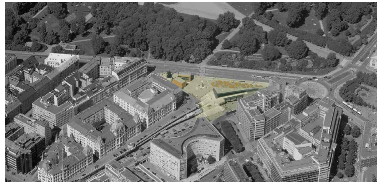
Fig. 18. Selected building site, right beside the ministry of foreign affairs (Victorian building on the left).
