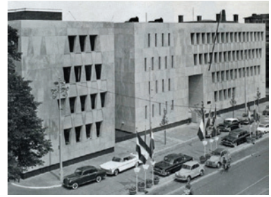
fig. 21; Plasticity in the façade and shading
