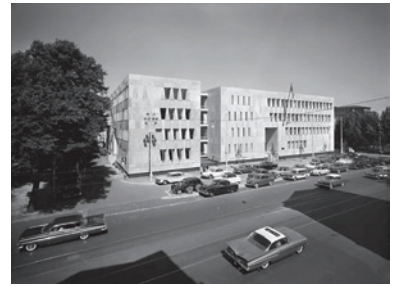
fig. 13; Analysis: Impression building U.S. Embassy after completion in 1959.
