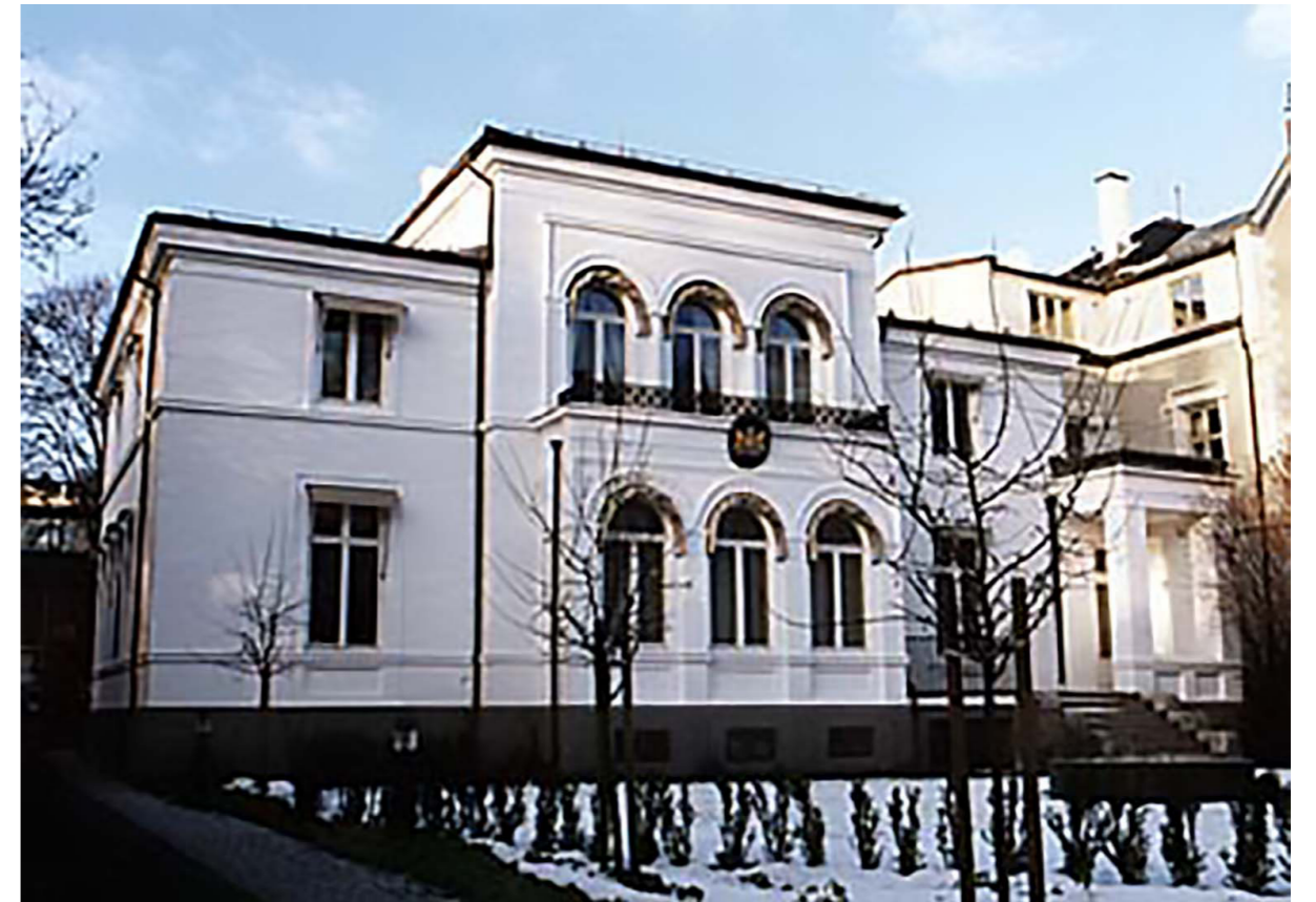
The Embassy building is located at Oscars gate 29 in the Homansbyen district. The architect of the original house was Wilhelm von Hanno.
