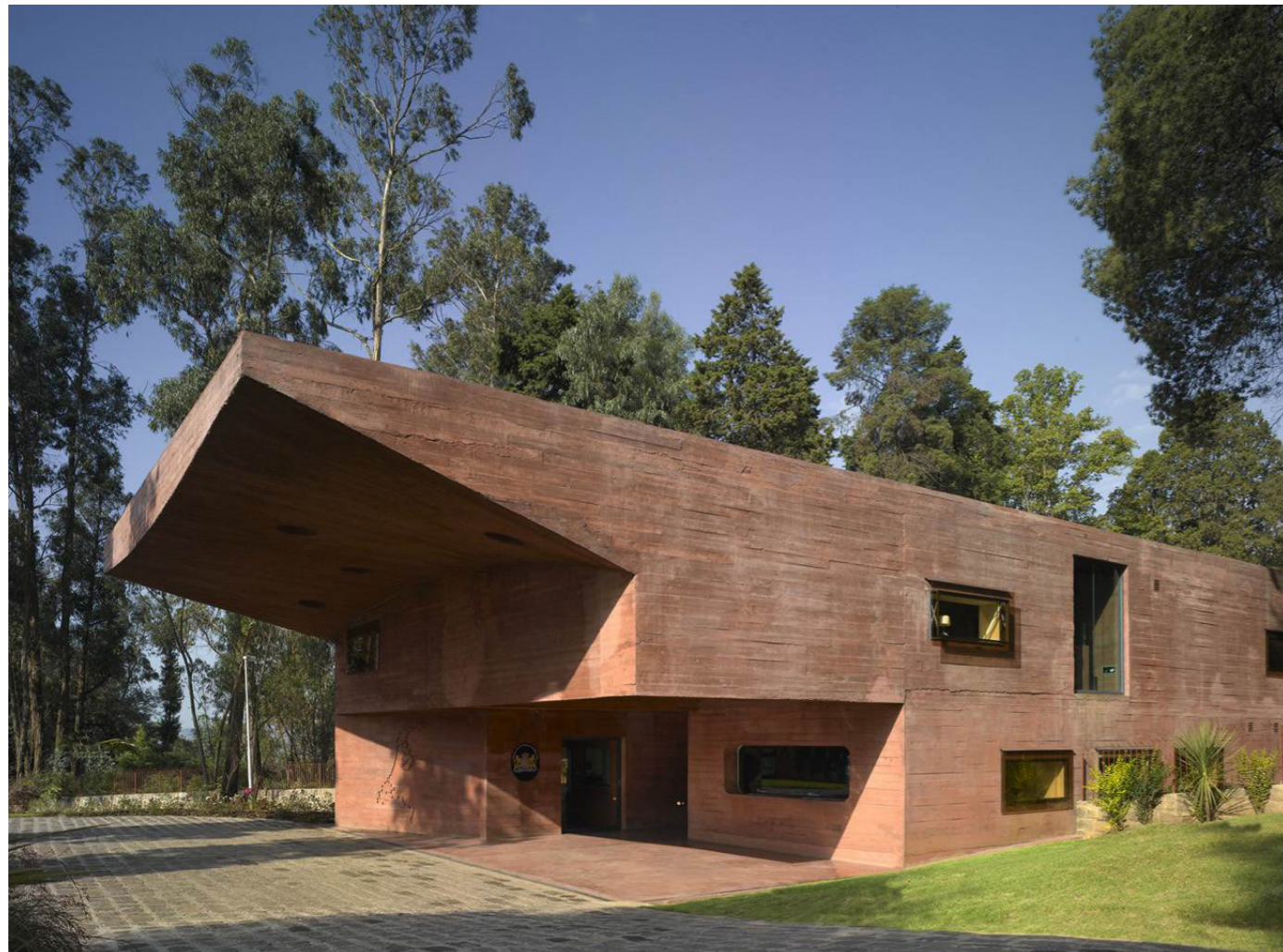
The main entrance has a strong jutting cantilever
