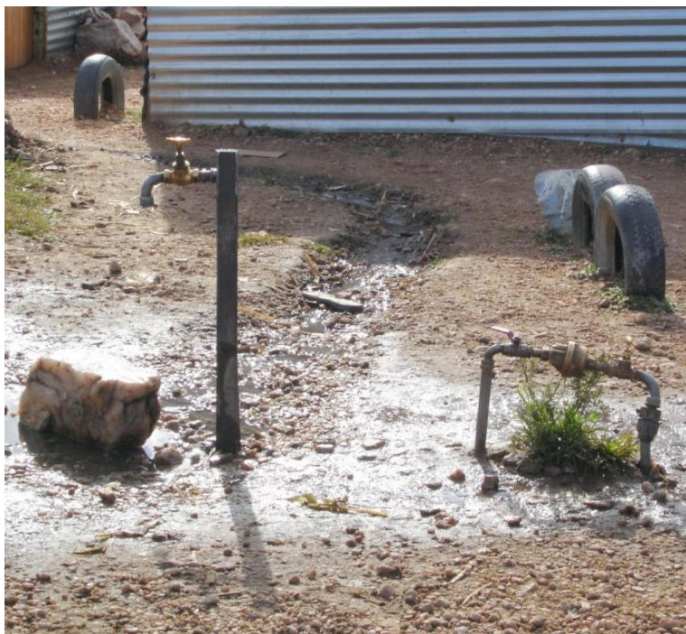
Figure 6: A communal tap with conventional water meter on the right (Kastner, McHugh, St. Martin, & Youssef, 2005).
