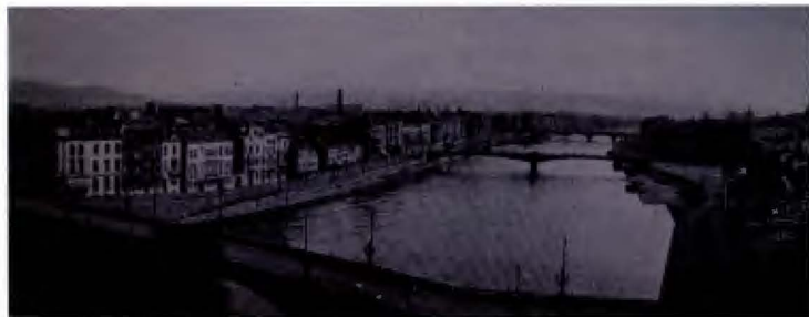
FIGURE 27. PANORAMA OF THE MEUSE AS SEEN FROM THE EAST
