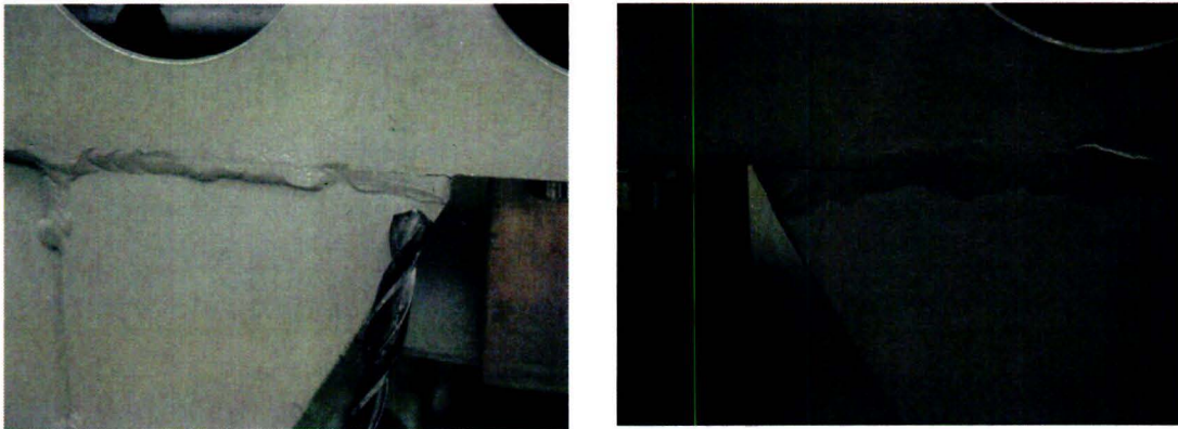
Figure 2.6.2 Cracked aluminium welds
