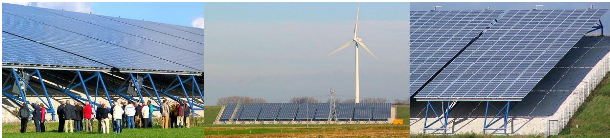
Figure 23: PV park at the slope of a landfill site in Waalwijk, the Netherlands.
