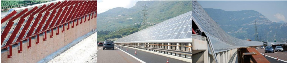
Figure 21: 730 kWp PVNB in Marano, Italy.
