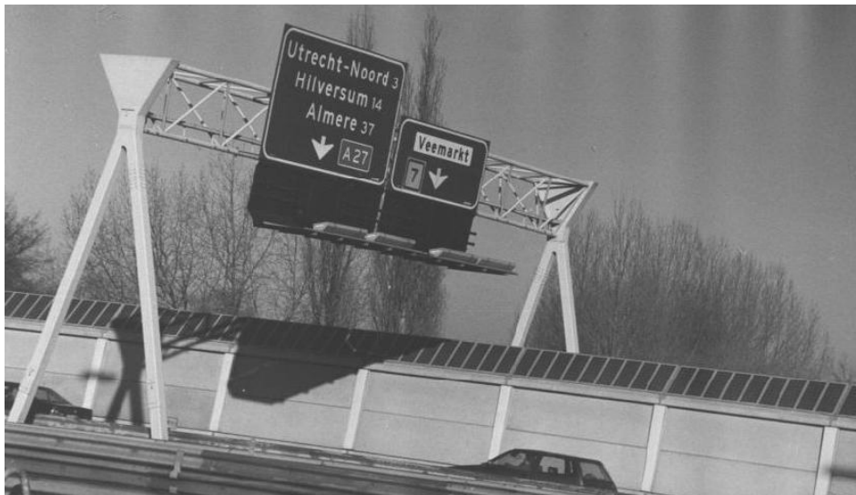
Figure 27: Shadowing of a sub array caused by the road signs along the A27 (Betcke et al., 2002)
