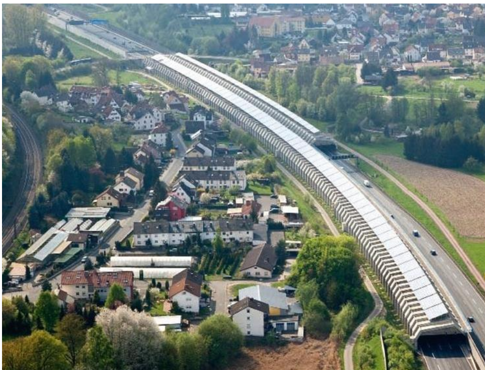
Figure 22: Solar array on the tunnel near Aschaffenburg, Germany.
