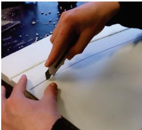
Figure 7.18: Cutting slices in the XPS formwork
