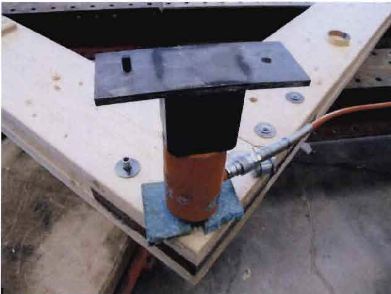
Figure 78: Placement of protection to prevent launching of the rod due to rod failure
