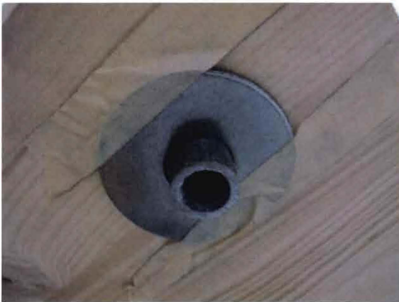
Figure 72: Placement of lower ring
