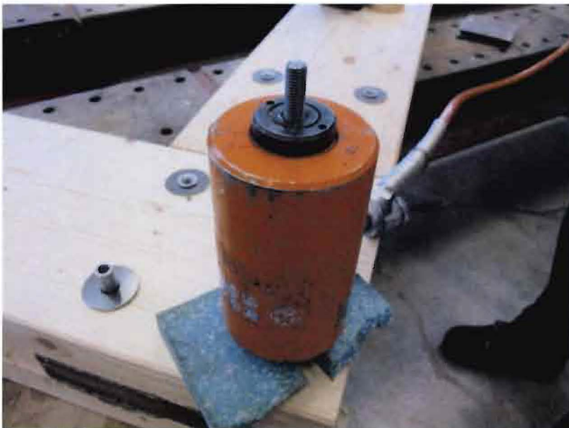
Figure 76: Placement portable hydraulic jack
