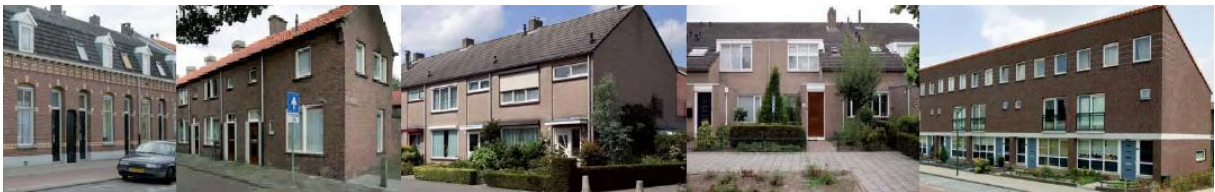
Figure 3.6: Terraced houses from five building periods (AgentschapNL 2011)
