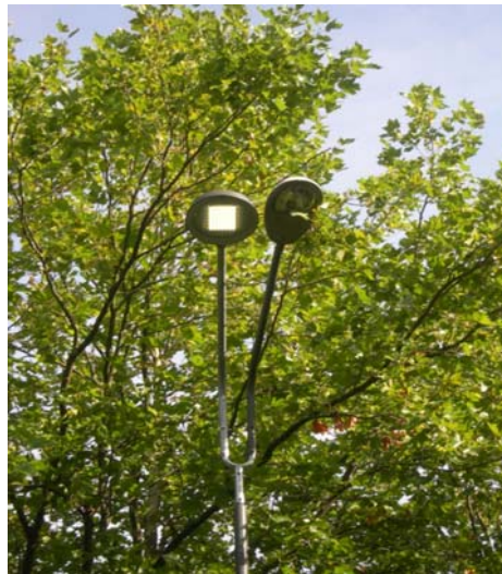
Figure 2. Road lighting lamppost equipped with both led unit (working) and high pressure sodium lamp
