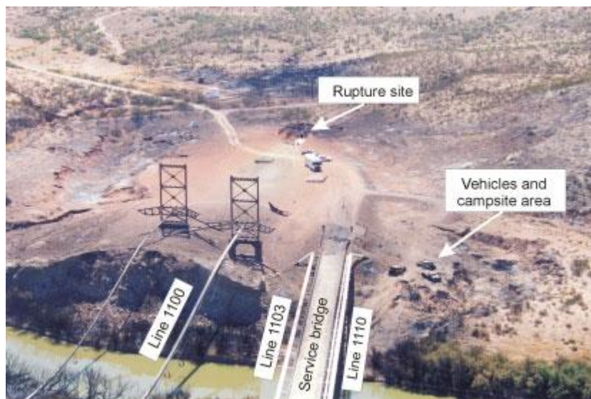
Photo 11: Aerial view of accident site looking east.
