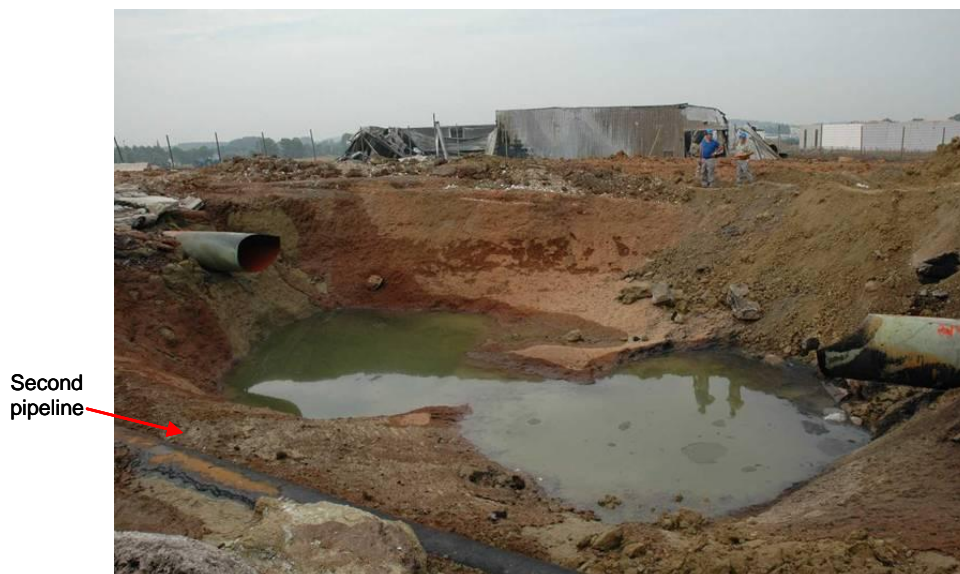
Photo 6: Crater from the pipeline rupture, (Belgium Min. Econ. Aff.)
