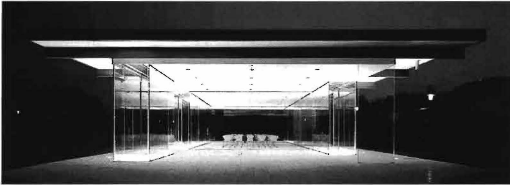
Figure 1.1 A structural challenge: dematerializing that part of the building that is responsible for keeping it up. In the Rheinbach Glass Pavilion –designed by Jörg Hieber and Jürgen Marquardt– the entire roof supporting structure is made of glass [Wellershoff and Sedlacek, 2003] which results in a seemingly floating roof structure. The structural safety concept is based on a combined probabilistic and consequence-based approach.
