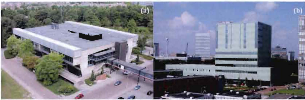
Figure 2.5: Photograph of (a) the Auditorium and (b) the Vertigo building (Tue.nl).
