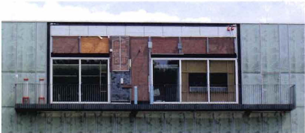
Figure 2.9: Photograph of the test facade of Vertigo.
