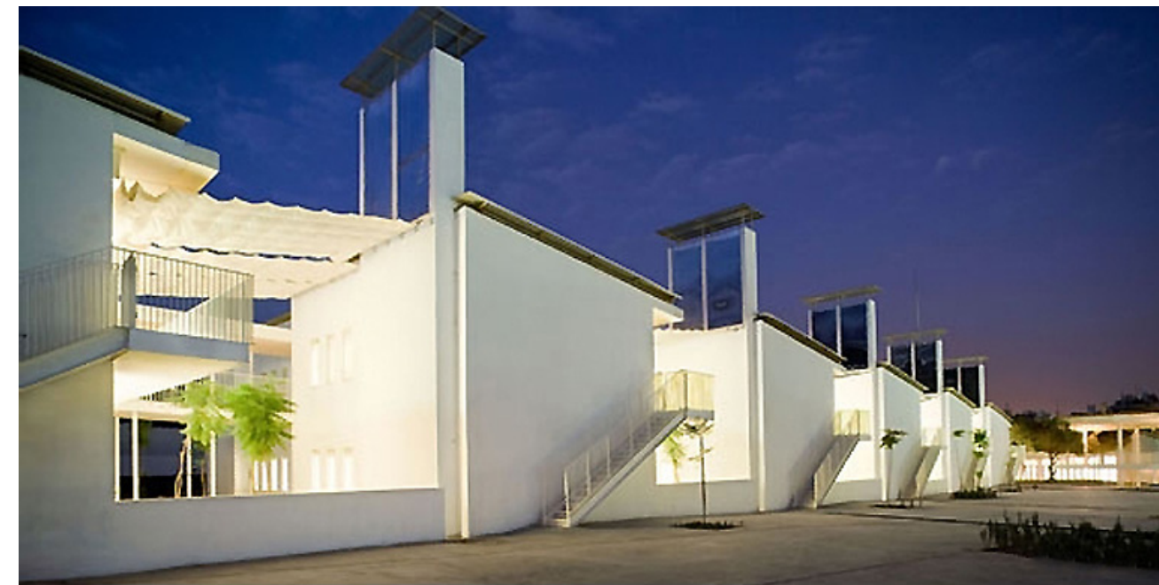
fig. 19 Lycée Charles de Gaulle (2008), by Ateliers Lion and Transsolar in Damascus, Syria. Solar chimneys are used to ventilate the buildings.
