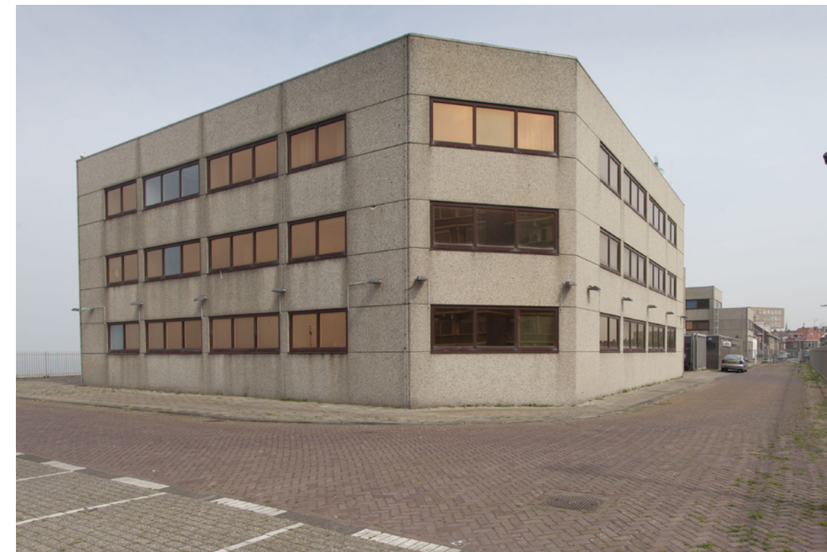
fig. 10 The building is clad in concrete facade panels with gold coloured glass.
