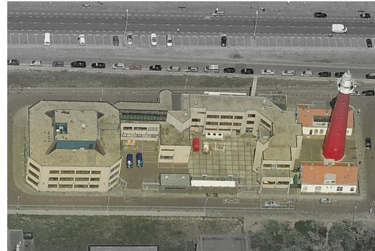
fig. 9 The former office building of the State Lighthouse office and the State Pilotage office is located on the coastal dyke at Vuurtorenweg, Scheveningen, The Hague.
