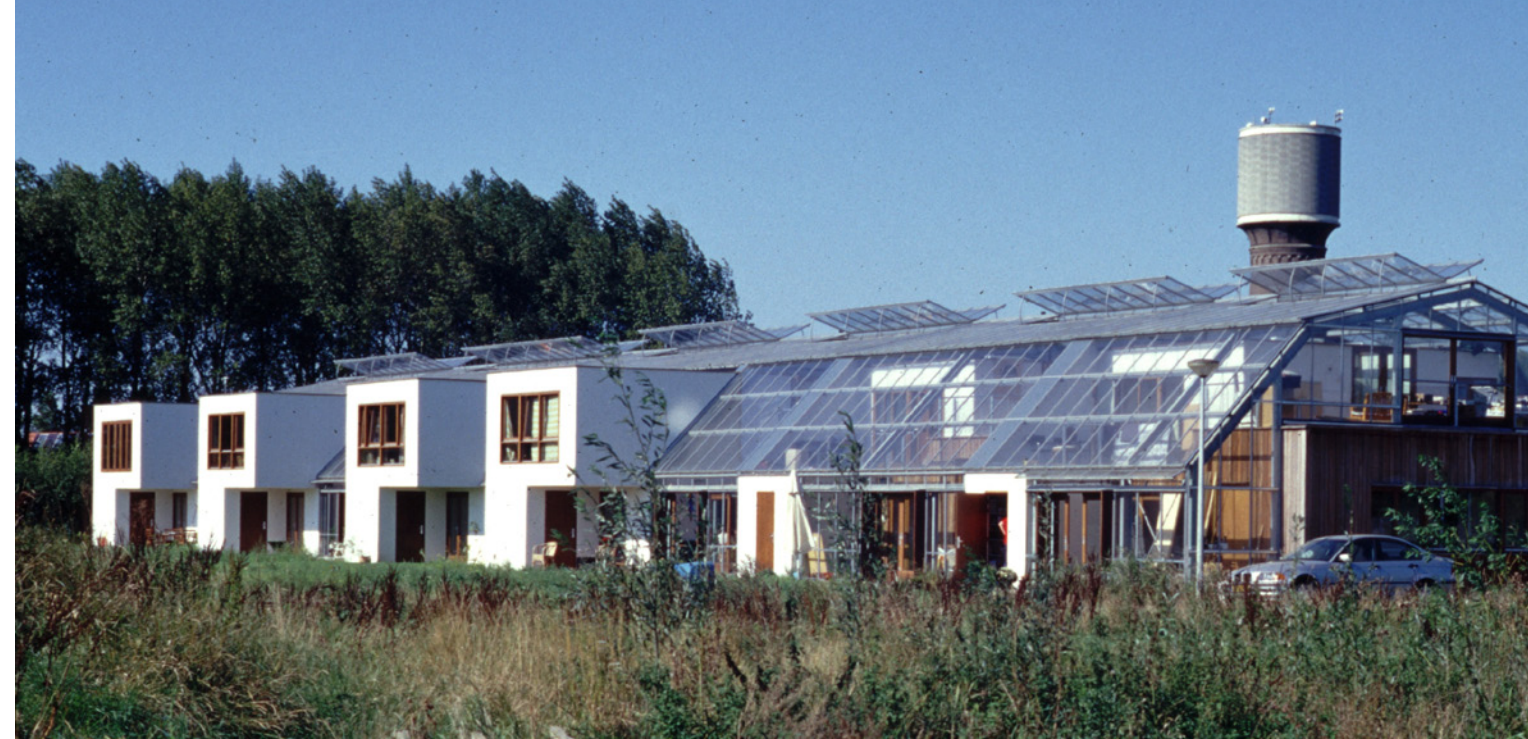
fig. 18 The 'greenhouse houses' (2009) by KSWA architects in Culemborg include a greenhouse-like atrium which creates a buffer between inside and outside. In cold seasons, the atrium is heated by the sun to provide a warm semi-outdoor space. In summer, sunshading protects the atrium from overheating.
