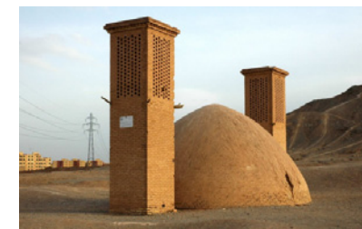
fig. 15 Building for hot climates: wind towers in Yazd, Iran
